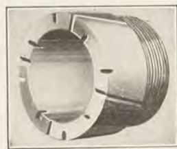
FIG. 159.—Diamond drill bit.
