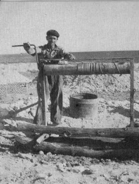
• This miner is hauling a bucket to the surface while his partner works below ground level. An empty bucket is seen in the background.
