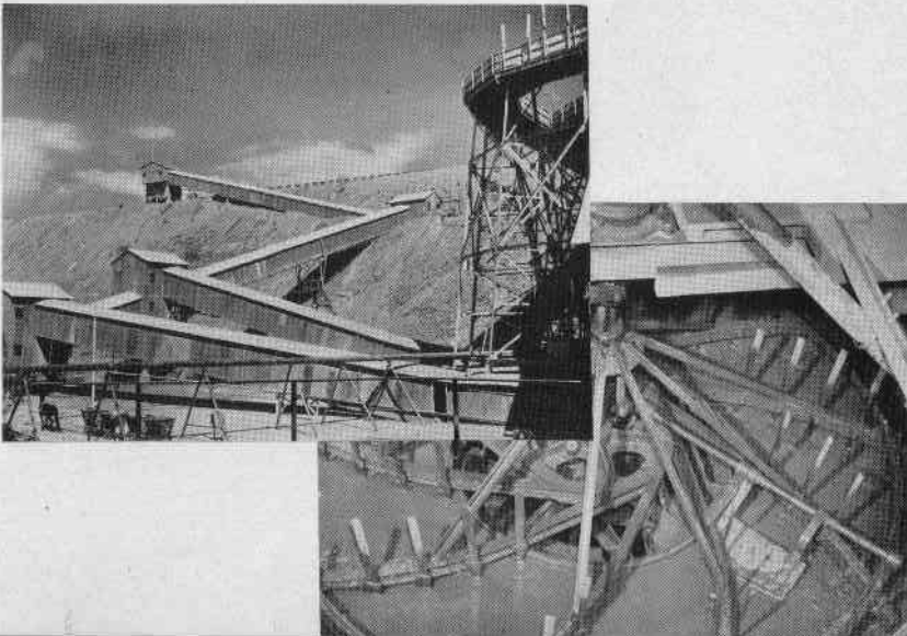
● The Shaft Head Frame of the Hoist Engine House of Dutoitspan Mine as it appears today. The shaft head frames are 115 feet high.
