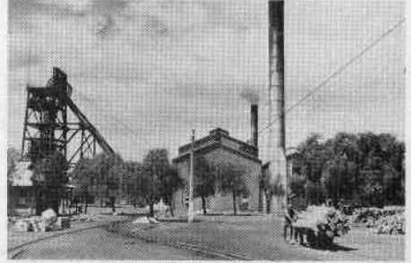
● The Shaft Head Frame of the Hoist Engine House of Dutoitspan Mine as it appears today. The shaft head frames are 115 feet high.
