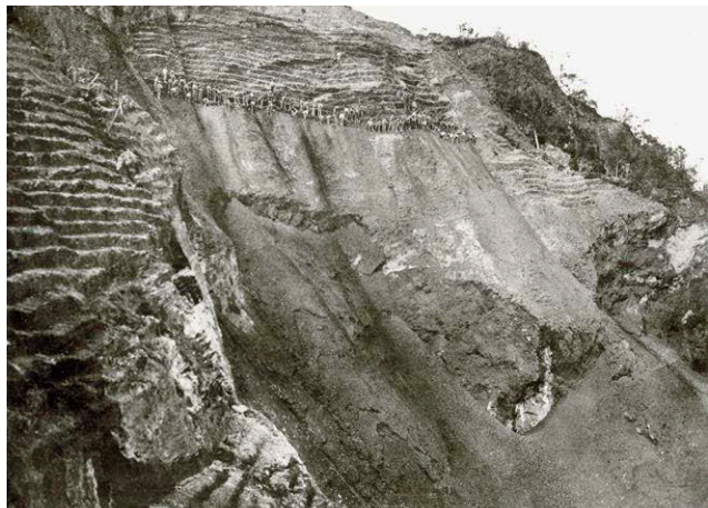
Figure 26. Mining at Chivor in the 1920s was performed exclusively by the open-cut method, preparing terraces or narrow steps in the extremely steep environment. Indigenous miners worked with long iron bars and hoes to remove the overburden and locate emerald-bearing veins or cavities. Photos of open-cast mining at Banco Klein, circa 1920 to 1921, courtesy of Carola Kroll.
