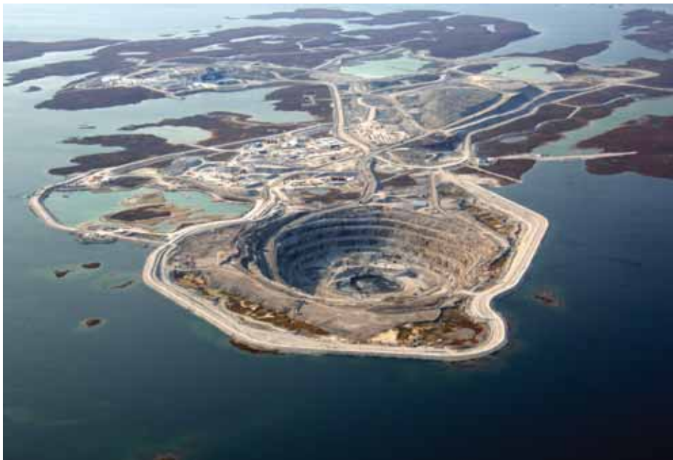
Figure 13. Canada's dramatic rise up the rankings in world diamond production has been the result of rich mines such as Diavik, shown here in a September 2006 image. A large dike had to be constructed to hold back the waters of Lac de Gras and allow safe open-pit mining of the A154 South and A154 North kimberlite pipes in the foreground. Just left of the A154 open pit, work has begun to expose the A418 pipe; production from that pipe is expected to begin in late 2007 or early 2008. Photo by Jiri Hermann, courtesy of Diavik Diamond Mines Inc.
