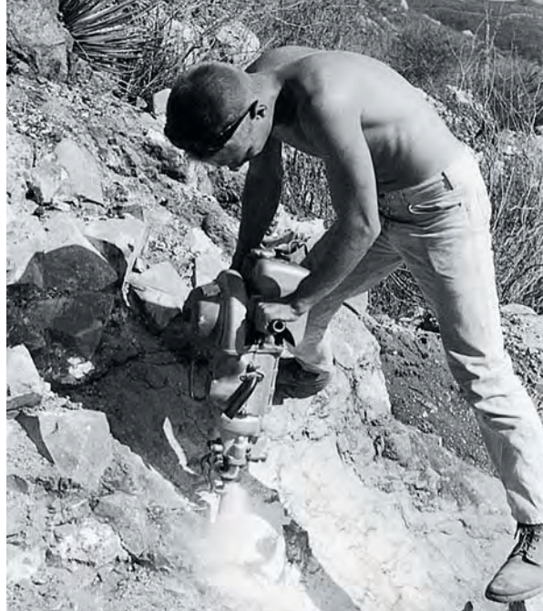
Figure 6. The Hercules dike was mined for spessartine by John Sinkankas and his son John William Sinkankas in the mid-1960s. This photo shows Sinkankas Jr. drilling the pegmatite in preparation for blasting. Photo by John Sinkankas, February 1966.
