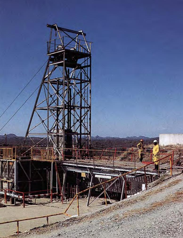
Figure 6. The main production shaft at the Zeus mine, the No. 3 shaft, serves as a haulage shaft down to 400 feet (122 m). Photo by E. J. Petsch.
