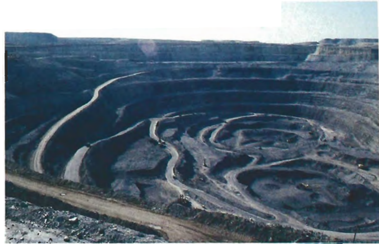
Figure 11. The Udachnaya kimberlite is currently the most important diamond-mining operation in Sakha. It is about 49 acres (20 ha; Johnson et al., 1989) in surface area. Large dump trucks remove the kimberlite and waste rock at a rate of about 1,000 metric tons per hour. The mine operates 24 hours a day and throughout most of the year.
