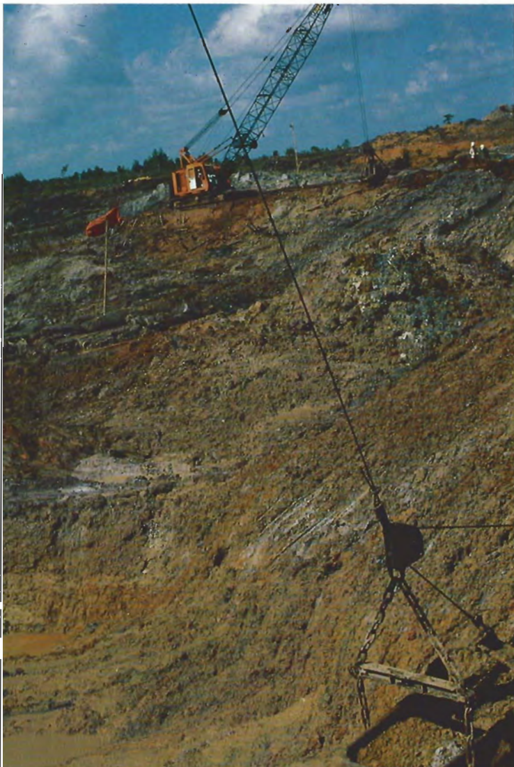
Figure 8. Clamshells are used to remove gravels from the first sample pit at Danau Seran. Photo by David Dikinis.
