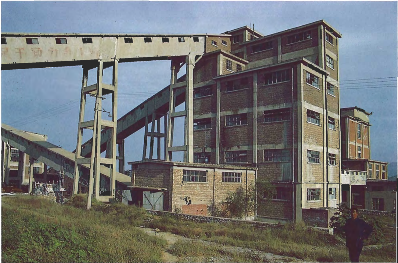
Figure 7. The diamond treatment plant is adjacent to the Victory No. 1 mine. The plant, which has been in operation since 1975, processes about 120 tons of kimberlite ore each day.
