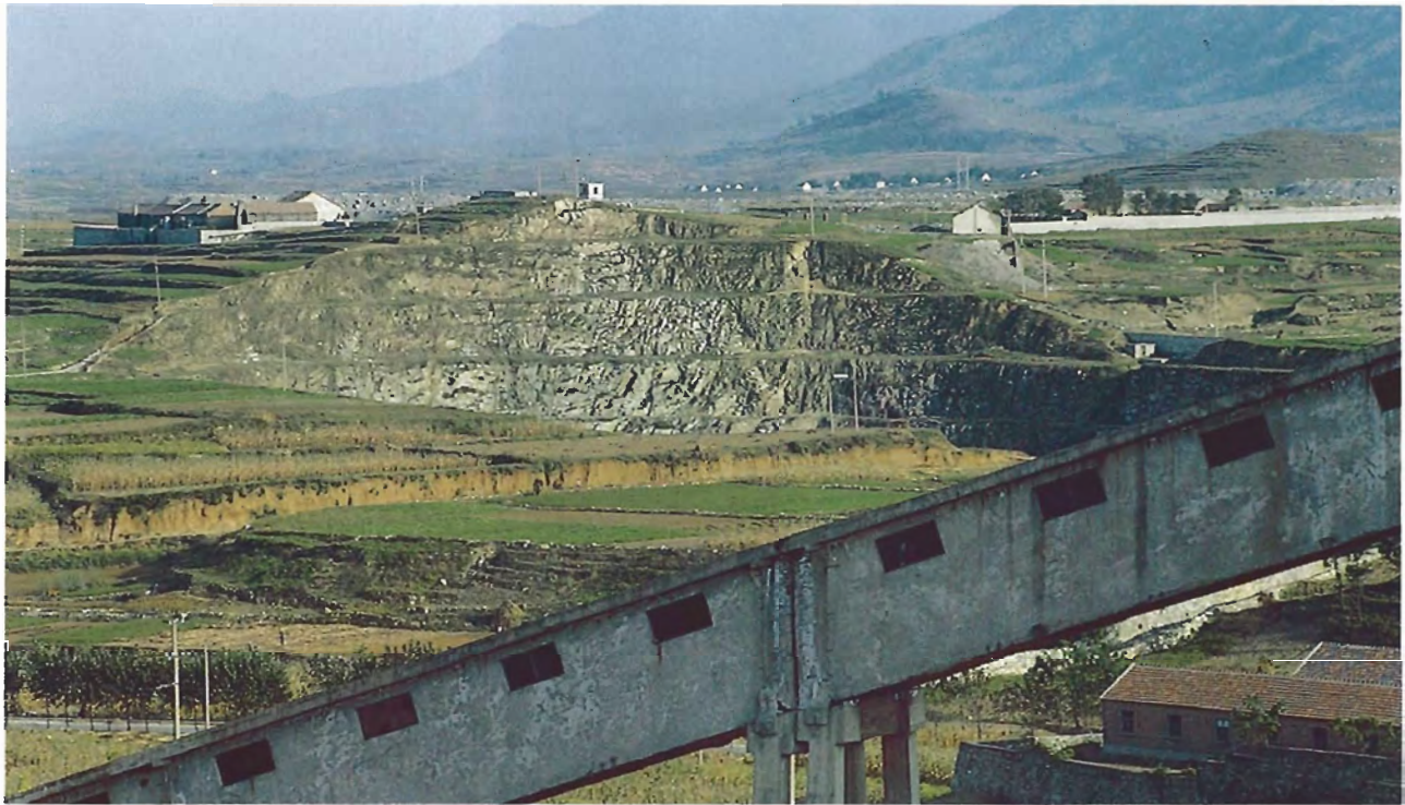
Figure 2. A view looking west toward the Victory No. 1 open-pit mine. The structure in the foreground is a portion of the diamond treatment plant constructed in 1975.
