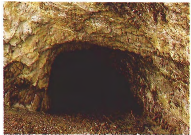
Figure 5. Low tunnel dug into metamorphic rock to reach the deeper mafic rock (note the white bands of magnesite).
