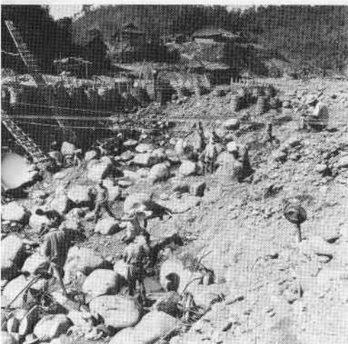
Figure 8 Stream-bed workings along the Uru. The majority of the boulders lying about are waste. The chicken ladders to the left carry waste material onto the dam that separates the pit from the river. Jade boulders are stockpiled on the firm ground of the riverbank, in front of the miners' huts. The white wires spanning the pit designate the limits of the individual claims by the suspended and weighted cords that reach the floor of the mine.
