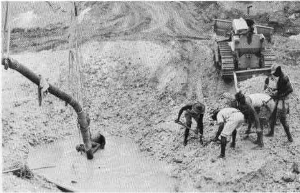
Tractor used to haul out gravel for treatment.
