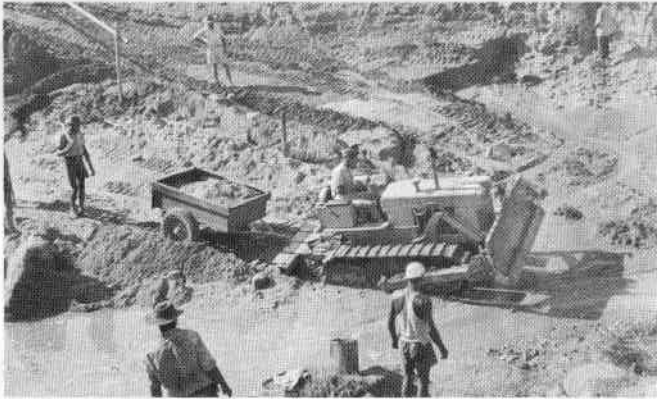
Tractor used to strip off overburden.
