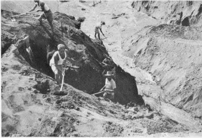
Ground sluicing off the overburden.
