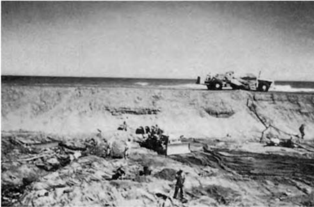
Figure 2.13 Removing the overburden of sand to recover diamond-rich gravels along the desert coastline of Namibia in South-West Africa. (Courtesy of De Beers)
