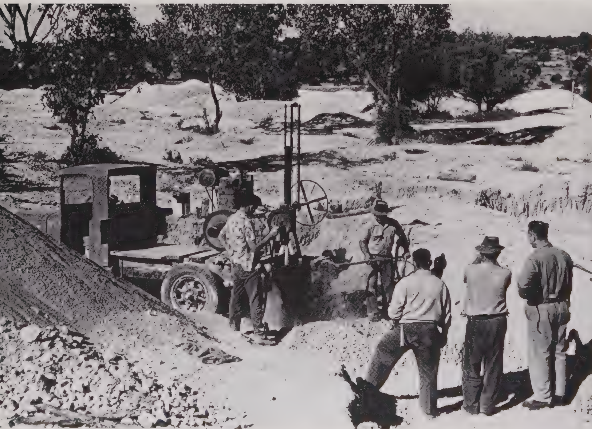
OPPOSITE BOTTOM: Visitors inspect "blower machine" which vacuums dirt from bottom of mine to surface, 1978 Photo: Joseph Ferdyn
