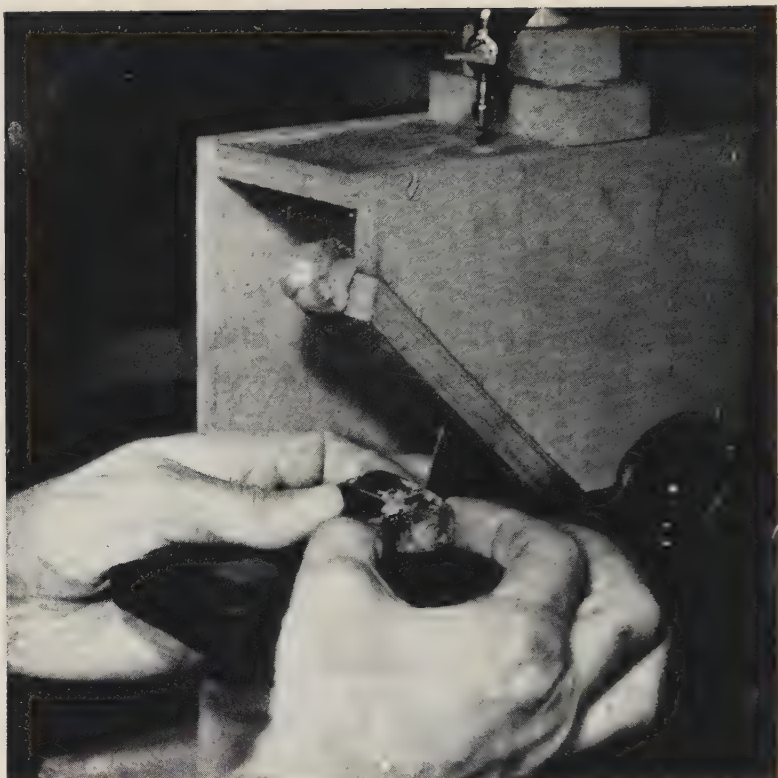
PLATE V. At work on the cut-off saw dividing a valuable gem crystal.
