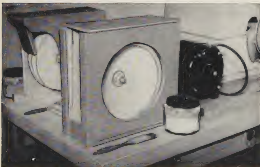
PLATE IV. Polishing bench, showing motor serving a double arbor with internal wooden polishing wheel and hard felt wheel.
