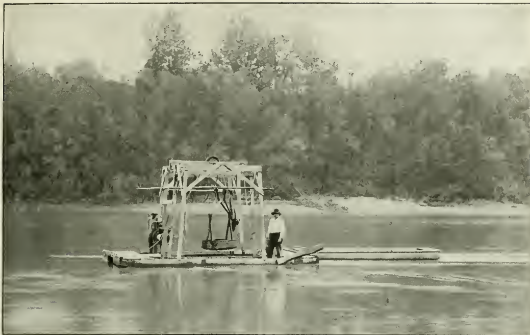
FIG. 1.—The dredge ready to be lowered into the water, Black River, Ark. (See p. 57.)
