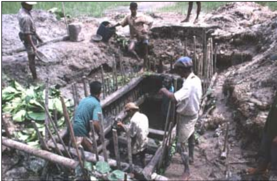
Plate 9: Initial headworks of a new deep gem shaft near Ratnapura
