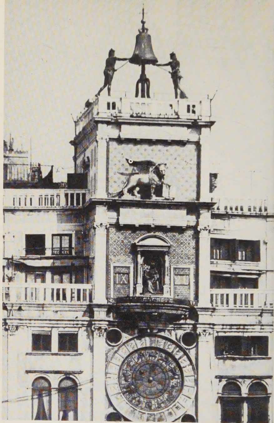
Clock tower of St. Mark's Square, Venice, showing the twenty-four hour dial and the jacks for striking the hours (see page 21)
