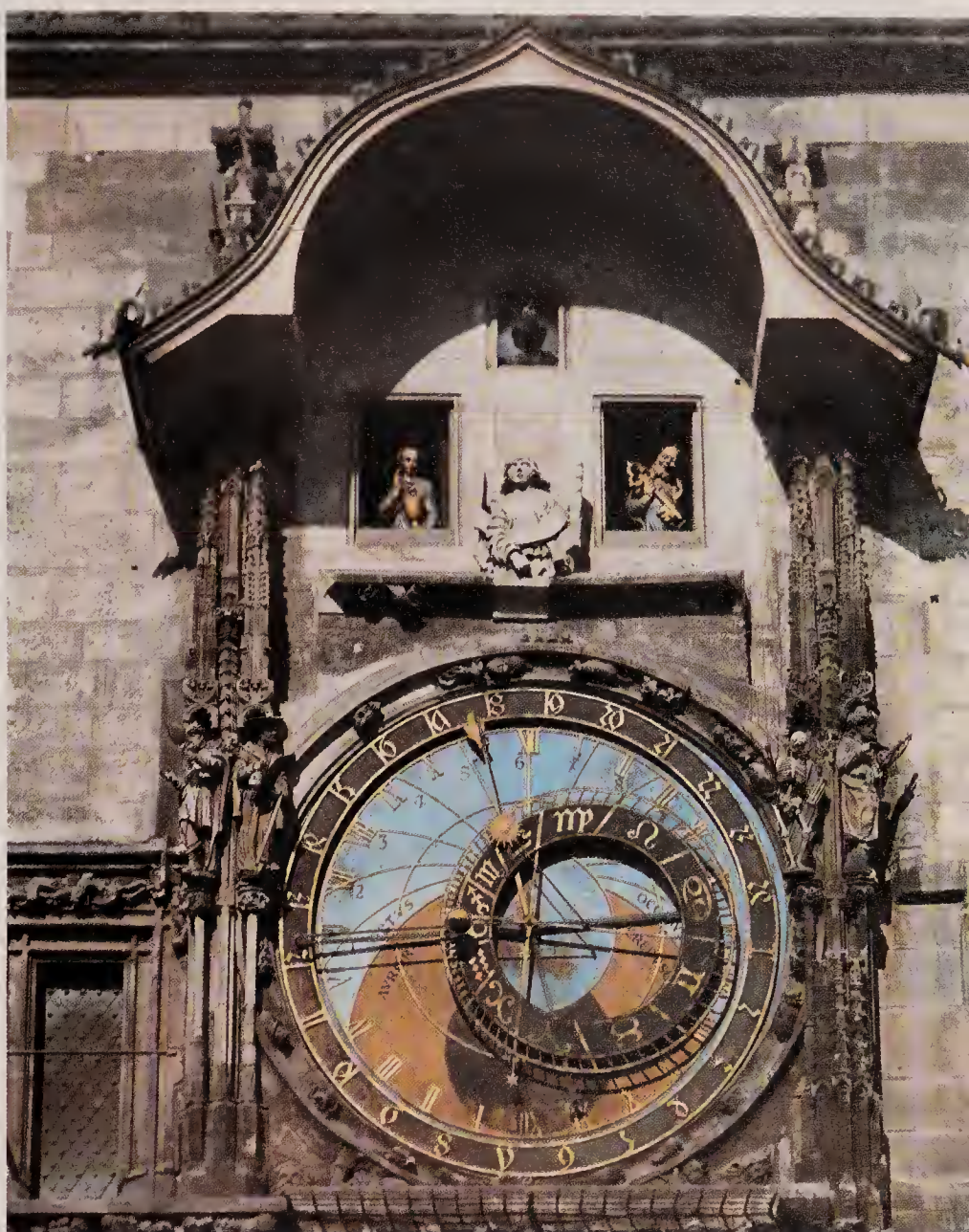
Above: The astronomical clock and automata at the Hotel de Ville, Prague. The original clock was built about 1486. Below is a calendar dial, and above, at the top of the tower, more normal dials which are driven by a separate movement.
