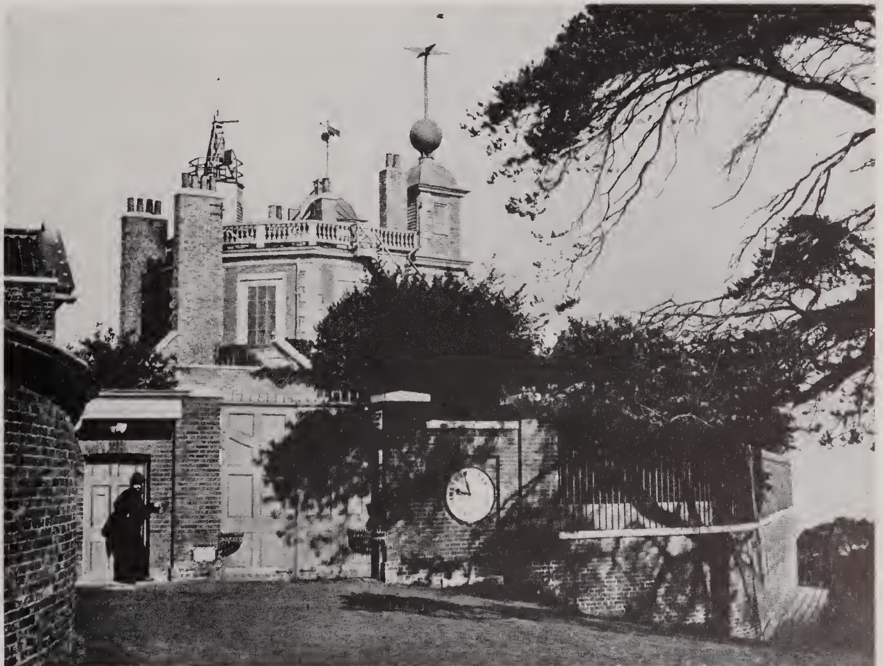
Right: Greenwich Observatory with Shepherd's clock, installed by Airey, and the time ball on the roof, which dropped at noon to signal time to shipping in the Greenwich Reach.
