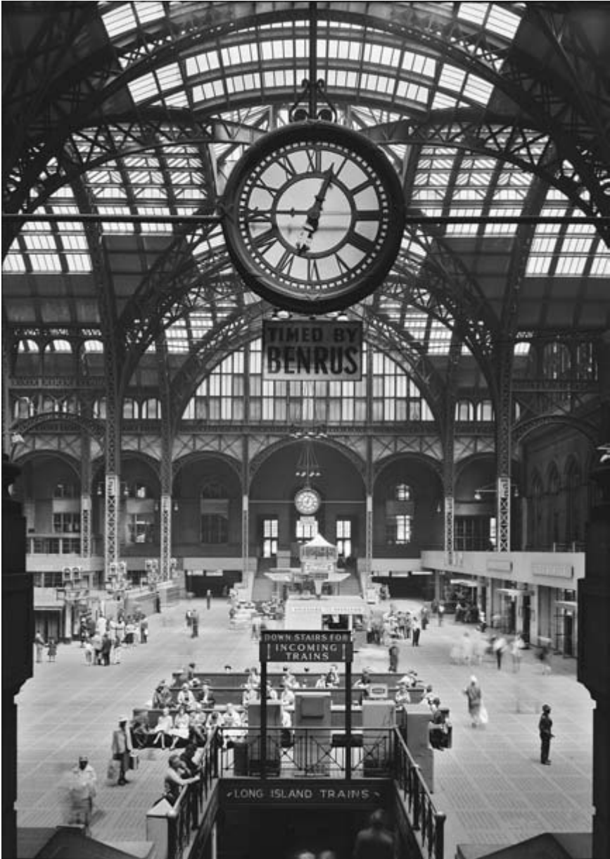
Cervin Robinson, Concourse from South , Pennsylvania Station, New York, April 24, 1962, HABS NY, 31-NEYO,78-79, Prints and Photographs Division, Library of Congress. Pennsylvania Station, home to an array of stunning public clocks, opened near Manhattan's center in 1910.
