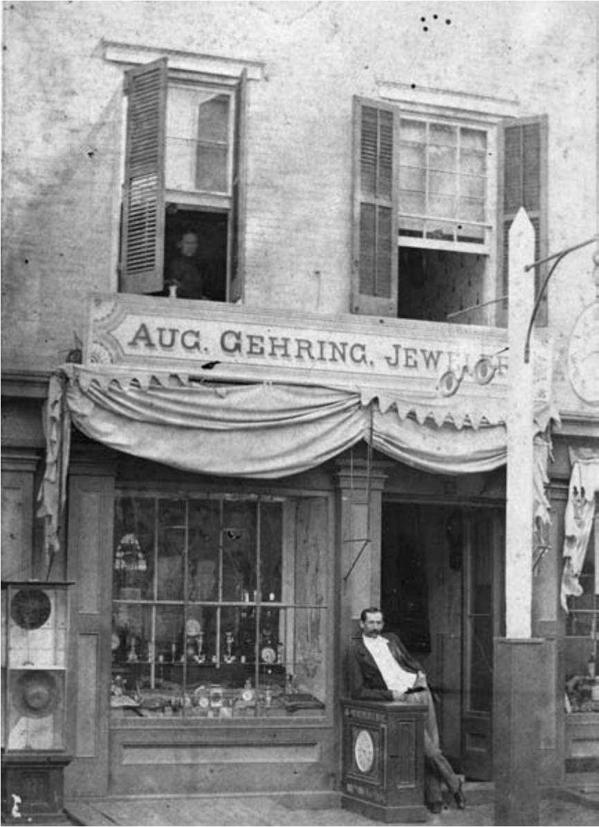
Storefront of Philadelphia jeweler Aug. Gehring, ca. 1880, photograph by A. W. Rothen-gatter and Company, courtesy of the Library Company of Philadelphia. An early version of the street clock was a double dial affixed to a post. The tubing through which the dials were attached to a clock movement inside the shop is visible in this photograph.
