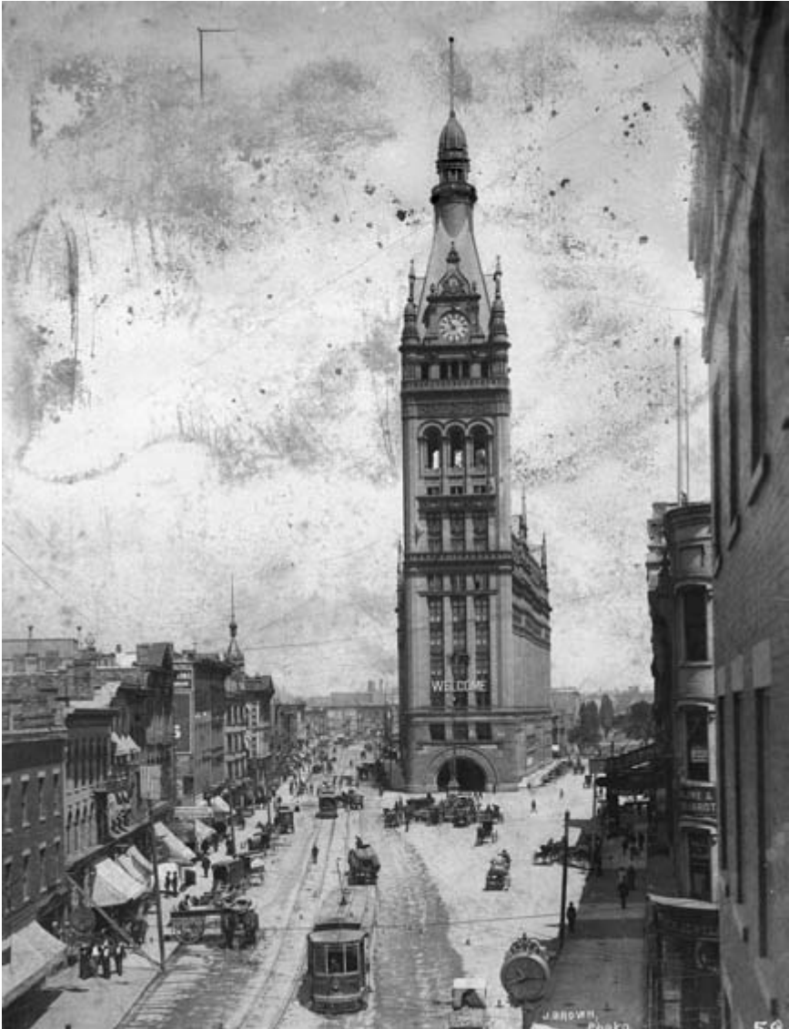
Milwaukee City Hall, 1904, WHI-48057, Wisconsin Historical Society. In 1896, when a tower clock was installed in the Milwaukee City Hall, it had the biggest clock face in the United States, with a diameter of fifteen feet. The large, heavy hands were so far from the clock room that a unique system using pneumatic tubes moved them. Warren S. Johnson, the same entrepreneur who would a few years later sell the city of Philadelphia its troublesome clock, designed it. The bell, weighing twenty thousand pounds, was one of the heaviest in the world: it took sixteen hours to hoist it into the tower.
