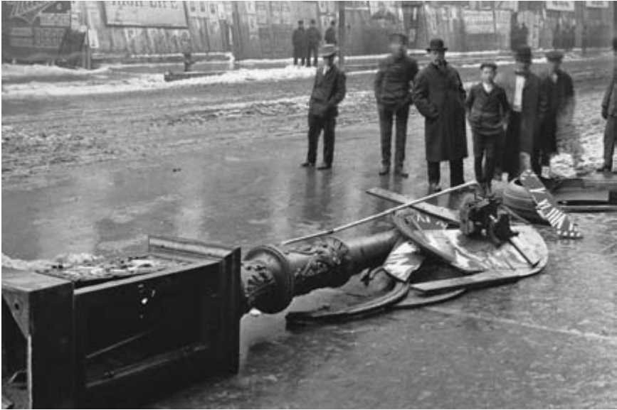
Destroyed street clock, Milwaukee, 1907, courtesy of Milwaukee County Historical Society. This was one among many photographs that dramatized the destruction of street clocks belonging to Milwaukee's jewelers.
