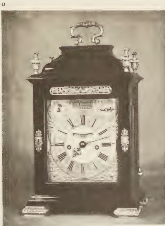
PLATE 57 Inverted-bell-topped bracket clock by Tompion and Banger, circa 1705-10. Note a strong general similarity to the earlier Tompion model, plate 51, and continued simplicity despite the increasing fashion for ornament. The back plate b is engraved with a conventional flowing pattern as against the tulip
