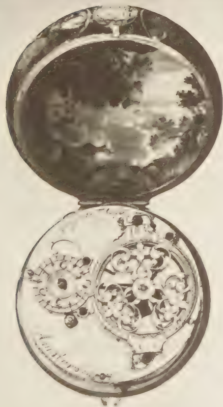
PLATE 79 Watch by Peter Paulus of Amsterdam with case painted in enamel on gold by the elder Huaud of Geneva. Late seventeenth century. a inside cover, b dial, c movement. (British Museum)
