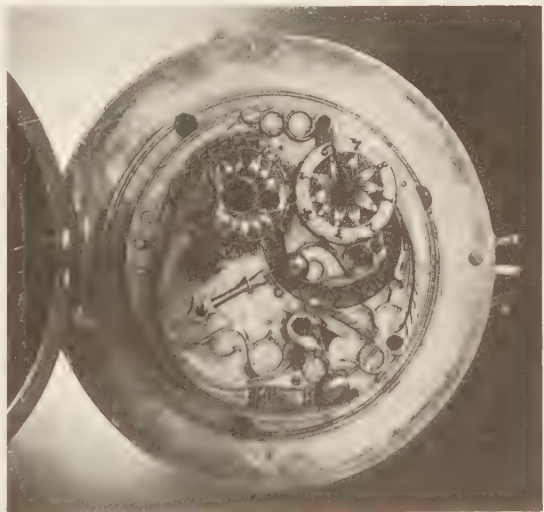
PLATE 17 Silver parcel-gilt crucifix clock. German. First quarter seventeenth century. Overall height 11 inches. a Brass movement in base drives a revolving chapter ring at the top of the cross. b The movement with bottom cover hinged open. Note stackfreed (in run-down position); count wheel with internally-cut gearing; foliot balance with bristle regulator operated by dial calibrated 1 to 8. (British Museum)
