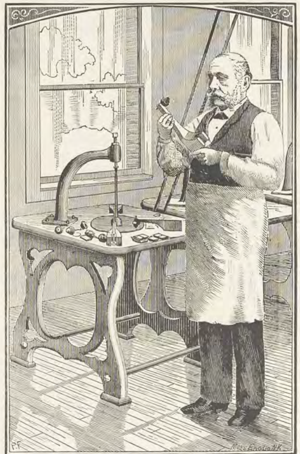
A PIONEER DIAMOND CUTTER—III. POLISHING.
