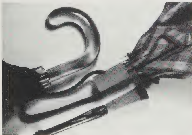
Figure 7.2 Umbrella handles in cast phenolic resin.
