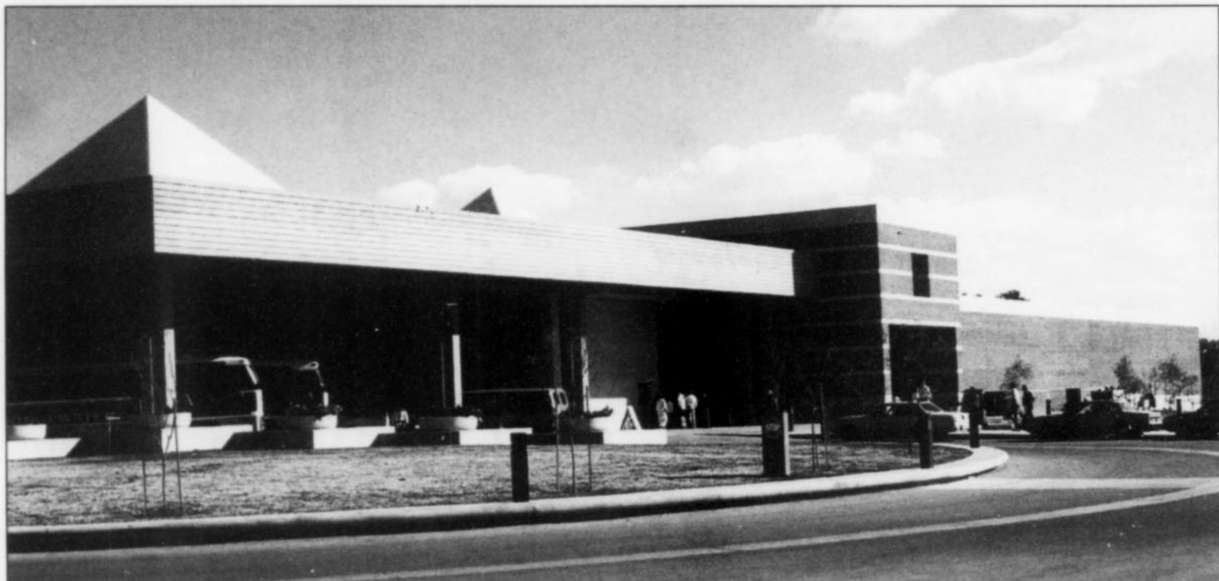
The newly built Tucson Convention Center took over as the site for the show in 1972 and expanded in 1989–1990 (Bob Jones photo).
