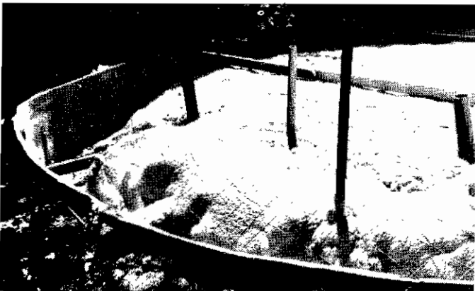
Formwork for foundation of 35 ft. diameter dome. Flexible plastic pipe is in place for use as conduits after slab is poured. The entire form was made in less than two hours of masonite and cable, covered with foam. Underneath the concrete slab is 1-1/2" of foam plus a polyethylene vapor barrier.
