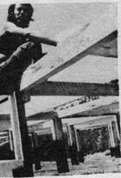
We stapled tarpaper over the joists and stringers and then laid 2 X 6" floorboards, alternating the direction of each 7 to 8 ft section so that the floor looks like a checkerboard. The tarpaper is to prevent drafts. Unfortunately, water collected between it and the boards while the floor was uncovered. It's probably still there.
