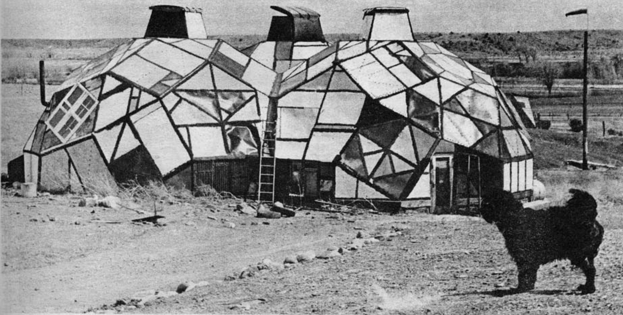
At left: Baer's fused triple rhombicosadodecahedra at Drop City, Colorado Below: Bill Chaitkin made this model from the Dome Cookbook of two fused rhombicosadodecahedra.
