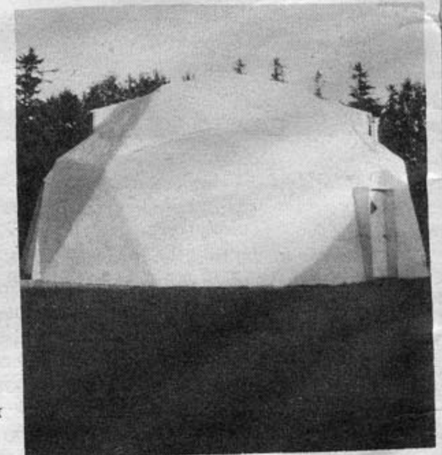
finished dome with white sealer
