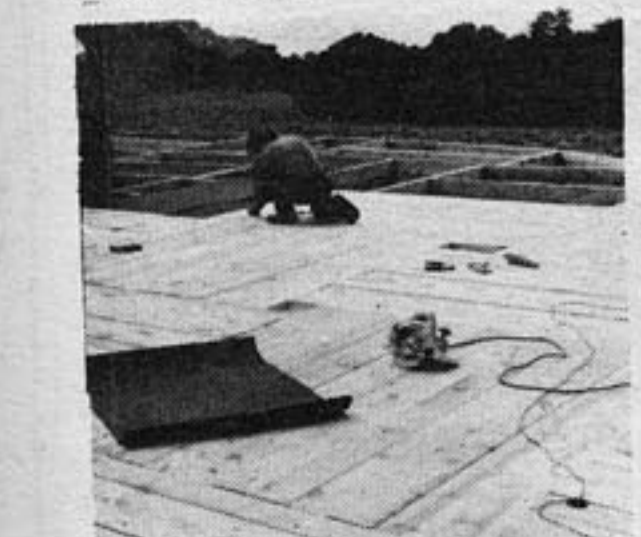
We stapled tarpaper over the joists and stringers and then laid 2 X 6" floorboards, alternating the direction of each 7 to 8 ft section so that the floor looks like a checkerboard. The tarpaper is to prevent drafts. Unfortunately, water collected between it and the boards while the floor was uncovered. It's probably still there.
