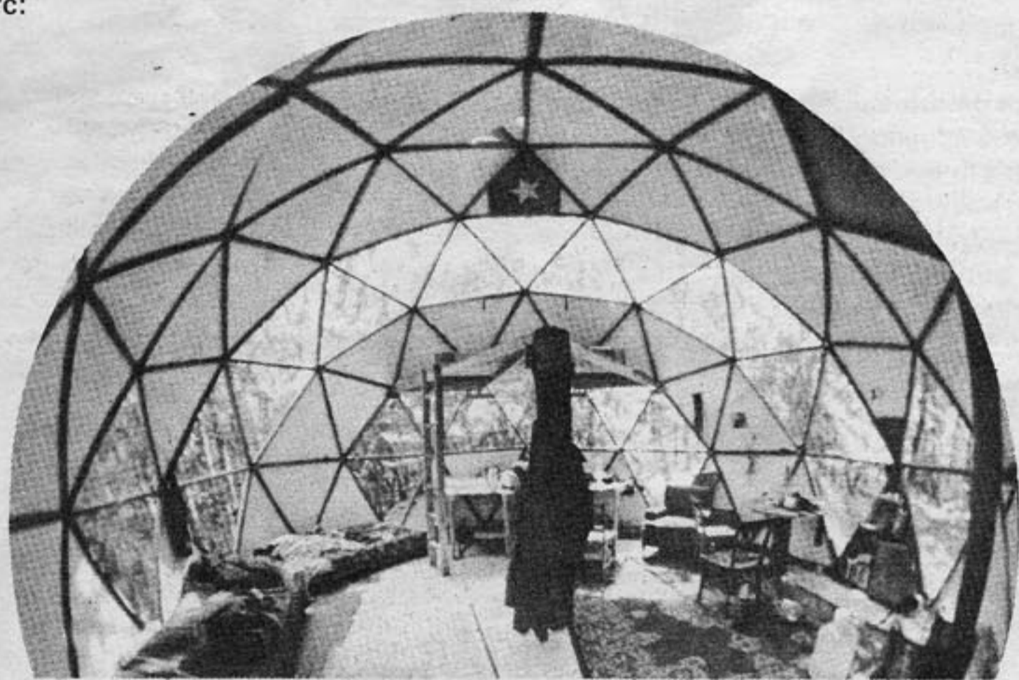
The 15-triangle arc was placed to correspond to the path of the winter sun.
