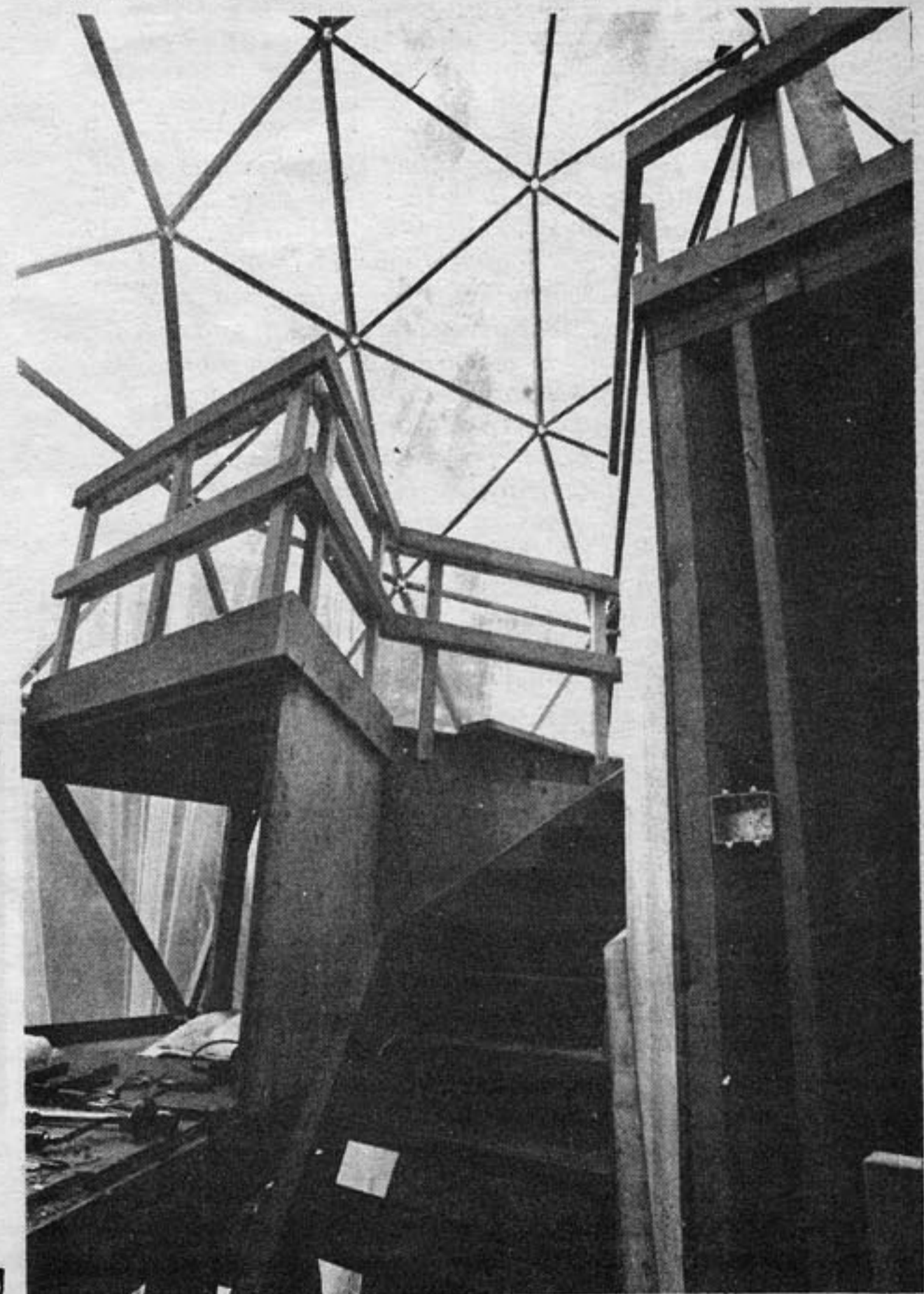
3/4 Dome temporarily covered with polyethelene bag
