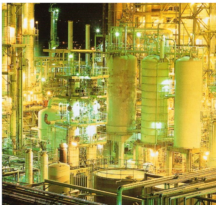
Plate 71 Crude Oil Oil refinery at night. At the refinery, crude oil is heated and passed through catalytic cracking towers. These are used to break up the heavy crude oil hydrocarbon molecules into lighter fragments. The resulting components, from heavy industrial oils and tars through to light fuels (such as petrol and kerosene) and gas, are separated out. The various components, called fractions, may then be collected and shipped separately. Photographed in British Columbia, Canada. (Reproduced with permission from Science Photo Library.)
