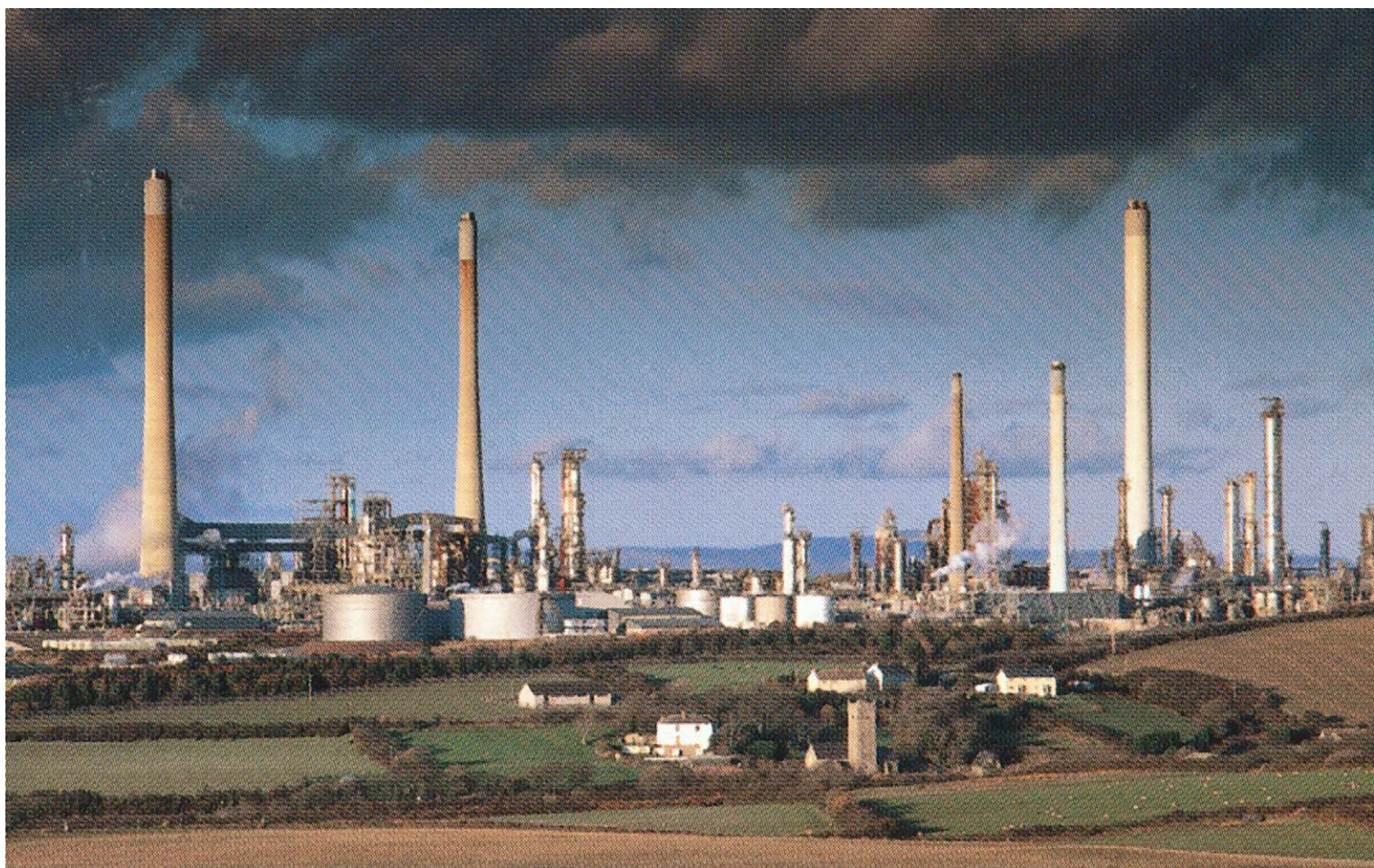
Plate 38 Distillation: Historical Development Oil refinery. Oil refinery with towers and chimneys. In an oil refinery, crude oil is heated and passed through catalytic cracking towers to break up the heavy crude oil hydrocarbon molecules into lighter fragments. The resulting components, from heavy industrial oils and tars through to light fuels (like petrol and kerosene) and gas, are separated out. The components, called fractions, may then be processed. Photograph of the refinery at Milford Haven, Wales. (Reproduced with permission from Science Photo Library.)
