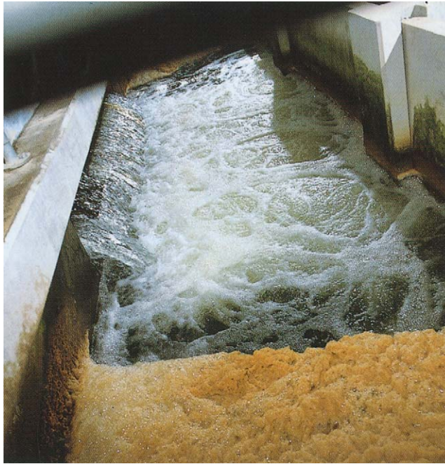
Plate 126 Water Treatment Waste water treatment. View of waste water entering a pool at water treatment plant. The water is undergoing a preliminary flotation separation process. Detergent foam (lower centre) floats on the surface of the water. This allows the waste water to be drained off and treated separately. Photographed in England. (With permission from Science Photo Library.)
