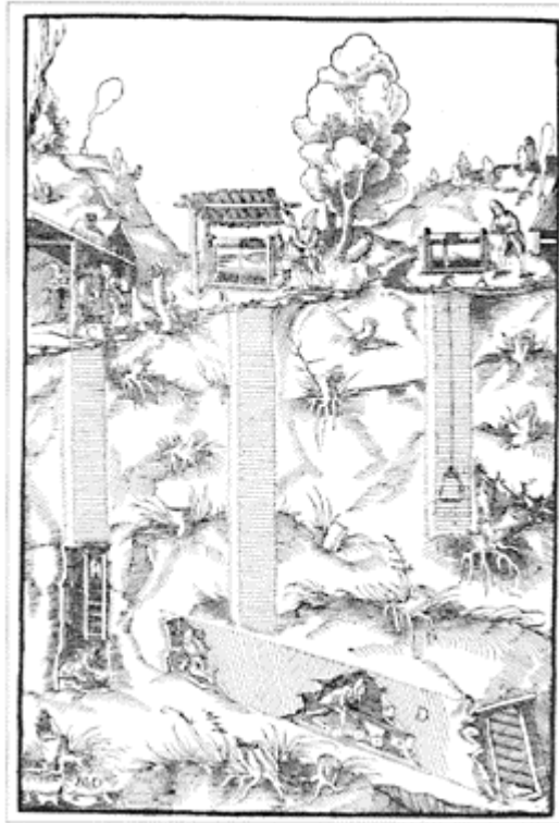
An illustration from Agricola's De re metallica (1556) showing three stages in the digging of shafts to create a mining tunnel.
