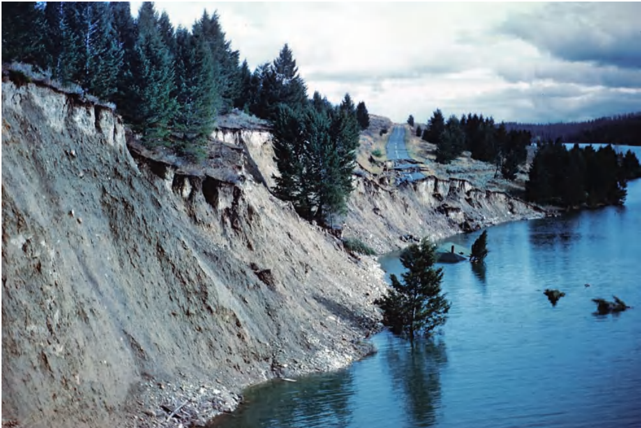
Slump of former State Highway 287 into Hebgen Lake, Montana, following an earthquake, August 1959 (USGS)
