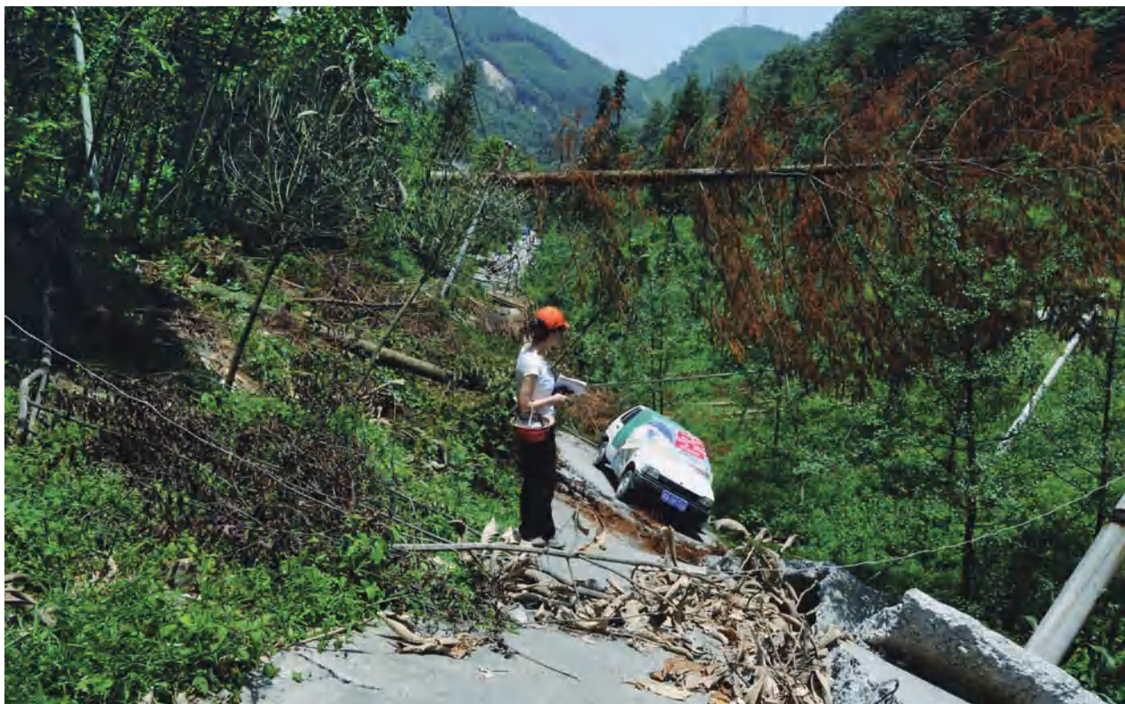
A second photograph of damage from ground shaking and landslides in Hongkon, Sichuan Province, China, from May 12, 2008, magnitude 7.9 earthquake ( T. Kusky )
