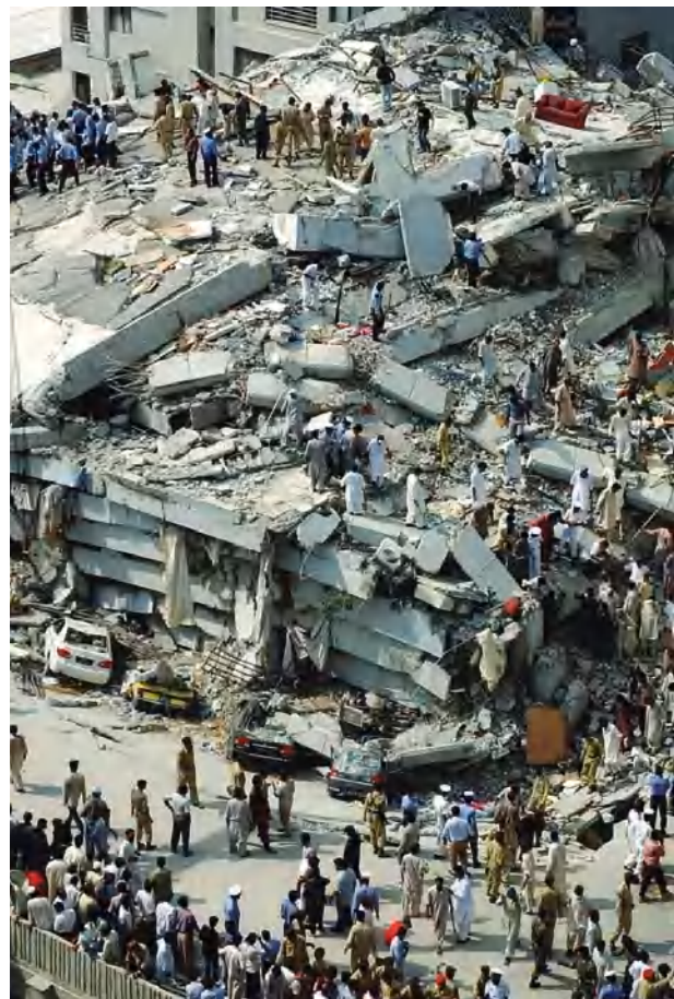
Collapsed 10-story apartment building in Islamabad, Pakistan, after earthquake October 8, 2005: The building pancaked as one floor fell, thereby causing each lower floor to collapse. (AP images)
