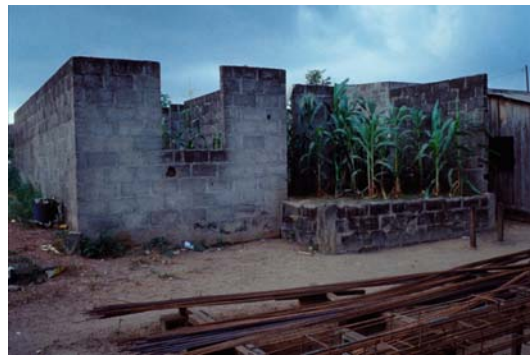
Cities and Towns in West Africa. Fig. 9 In a context of growing poverty, urban households turn to agriculture within and around urban areas in order to reduce their expenditures. Here, the Figure also shows the progressive building process in West Africa. Construction is usually incremental due to the underdeveloped nature of the housing finance system sector. Therefore, people build as they get money. © IRD – Philippe Haeringer.
