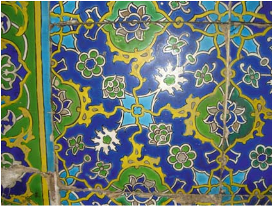
Architectural Decoration in Islam: History and Techniques. Fig. 16 Detail of cuerda seca tiles currently embedded in a re-constructed wall in the Topkapi Palace. Istanbul, Turkey. Late fifteenth century.
