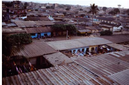
Cities and Towns in West Africa. Fig. 11 Abidjan, Côte d’Ivoire. Except in the downtown center and in some upper-class districts, the city skyline is very low and horizontal. 85% of the Abidjan population lives in compounds such as this. Several households surround the courtyard, usually the center of the plot. Each living unit normally comprises one room or two rooms of approximately 10 m 2 , one which is used as a bedroom and the other a sitting room. Three rooms is the maximum number of rooms for this type of housing and that is very rare. Courtyards are progressively filled with new constructions. At the rear, owners have started to build additional storeys. © IRD – Philippe Haeringer.
