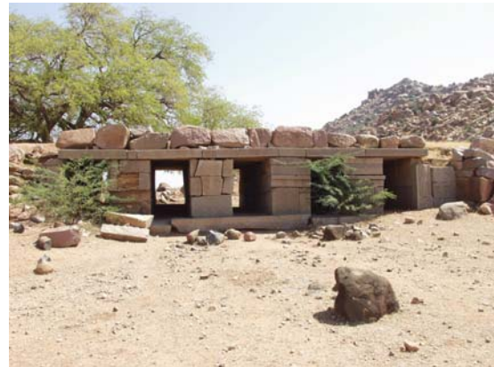
Water Management and Reservoirs in India and Sri Lanka. Fig. 6 Masonry waste weir, or spillway, to regulate high water levels at the edge of a Middle Period reservoir embankment near the village of Kurugodu (photo by Kathleen D. Morrison).
