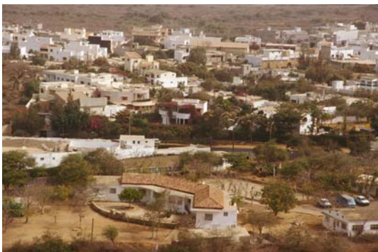
Cities and Towns in West Africa. Fig. 10 Dakar, Senegal. This neighbourhood is next to the airport area (rear of the Fig.). It was officially declared unsuitable for building development by the Senegalese government. However, this land was sold for construction by customary authorities of the Lebou (a local ethnic group). The quality of the houses shows quite well that unauthorized areas do not necessarily become slums. Nowadays, this type of neighbourhood is often regularized after construction (informal owners finally obtain titles from the public authorities). © IRD – Michel Dukhan.
