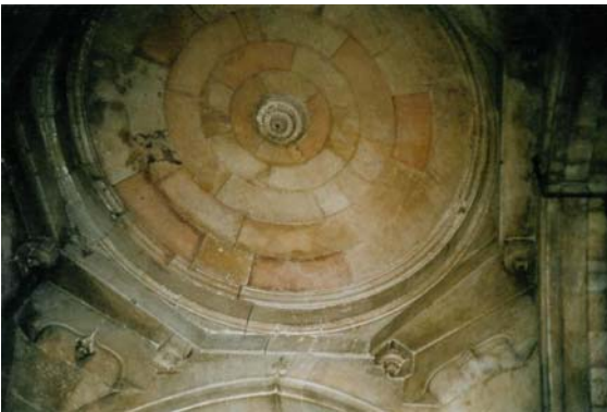
Building Construction. Fig. 12 Dome (Jumma Mosque, Ahmedabad). Ring forces balanced by overlapping; joints open where there is a little overlapping (photo by the author).
