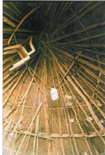
Building Construction. Fig. 9 Simple Bungha roof from the inside (photo by the author).
