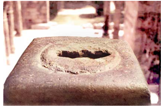
Iron Pillar at Delhi. Fig. 8 The top surface of the pillar capital presently contains a hollow slot.
