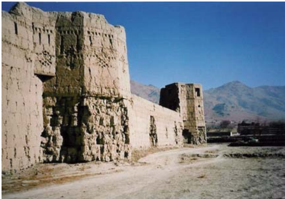
Building Construction. Fig. 4 Old castle near Kabul Afghanistan (with rammed earth) (photo by the author).
