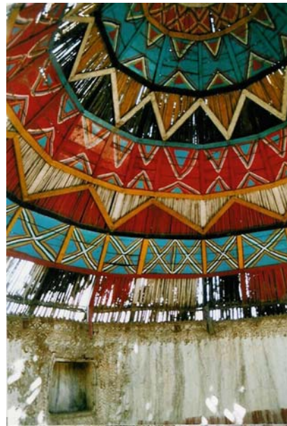
Building Construction. Fig. 20 Old Bungha roof (Kutch, Gujarat, India). Large roof without king post and excellent decoration (photo by the author).
