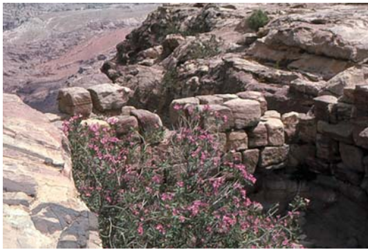
Water Management in Petra. Fig. 4 Elevated settling basin typical of the el Khubtha channel/piping system.
