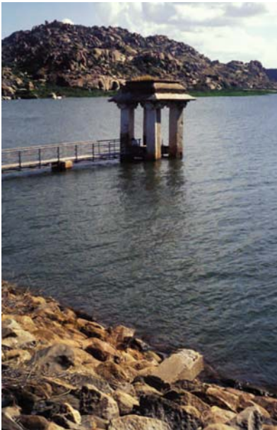
Water Management and Reservoirs in India and Sri Lanka. Fig. 5 The northern sluice of the Daroji reservoir, south of Vijayanagara. This “double sluice” construction became prominent in the sixteenth century, when the Daroji embankment was constructed. This sluice and reservoir have been maintained and continue to operate (photo by Kathleen D. Morrison).
