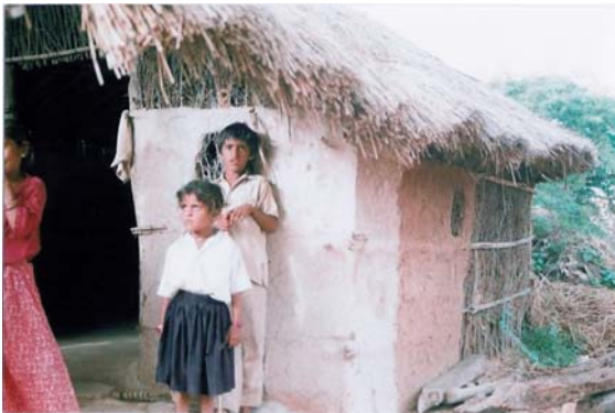
Building Construction. Fig. 1 Wattle and daub wall.
