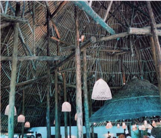
Building Construction. Fig. 11 Roof structure with tree-type supports (Beach Resort in Kenya) (photo by the author).
