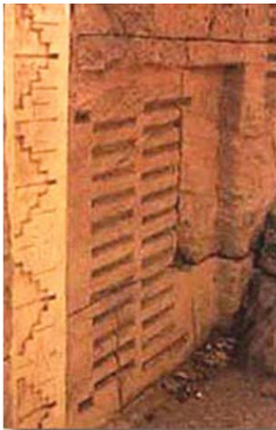
Nilometer. Fig. 9 (a) Staircase Nilometer at Elephantine: ▶http://www.lexicorient.com/egypt/aswan04.htm . (b) Close-up of the Elephantine gauge: ▶http://www.touregypt.net/featurestories/nile.htm .
