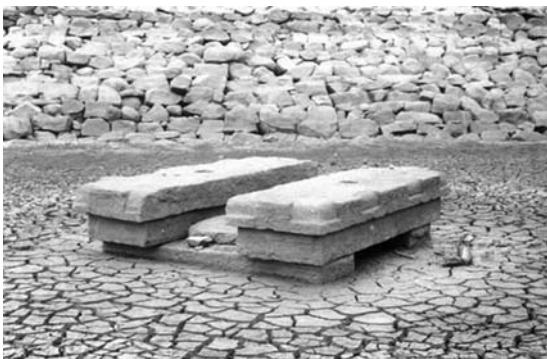
Water Management and Reservoirs in India and Sri Lanka. Fig. 9 Photo showing the accumulation of an estimated 2–3 m of silt and clay, to near the top of a sluice gate. This reservoir is adjacent to the village of Avinamodugu, south of Vijayanagara (photo by Kathleen D. Morrison).
