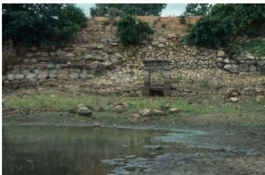
Water Management and Reservoirs in India and Sri Lanka. Fig. 7 Small Middle Period reservoir and sluice gate in the Daroji Valley, south of Vijayanagara (photo by Kathleen D. Morrison).
