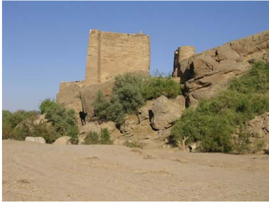
Dams and Irrigation in Ancient Arabia. Fig. 1 The massive south sluice of the ancient dam near Ma'rib, Yemen (photo by the author).
