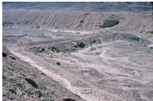
Water Management in Peru. Fig. 3 View of the low Hoya Hondada aqueduct across the wide quebrada. Photo by C. R. Ortloff.
