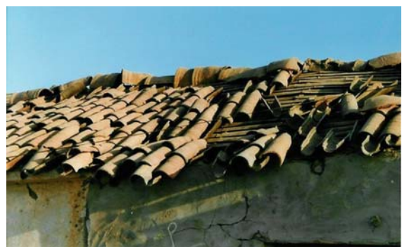
Building Construction. Fig. 13 Country tile roof (Gujarat, India). Split bamboo placed close together serves as battens (photo by the author).
