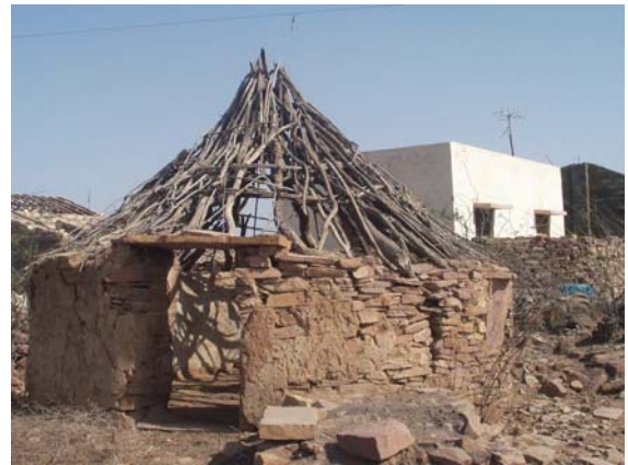
Building Construction. Fig. 10 A simple roof structure out of branches (Gujarat, India) (photo by the author).
