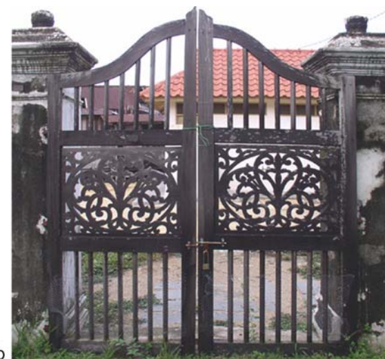
Woodcarving in Malay Architecture. Fig. 7 (a) A gate at Kota Lama Duyong for residents and neighbors. (b) A larger gate at Kota Lama Duyong for honored guests.
