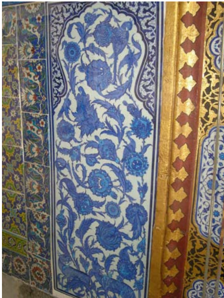
Architectural Decoration in Islam: History and Techniques. Fig. 17 Underglaze painted tile, Circumcision Room, Topkapi Palace. Istanbul, Turkey. ca. 1520.
