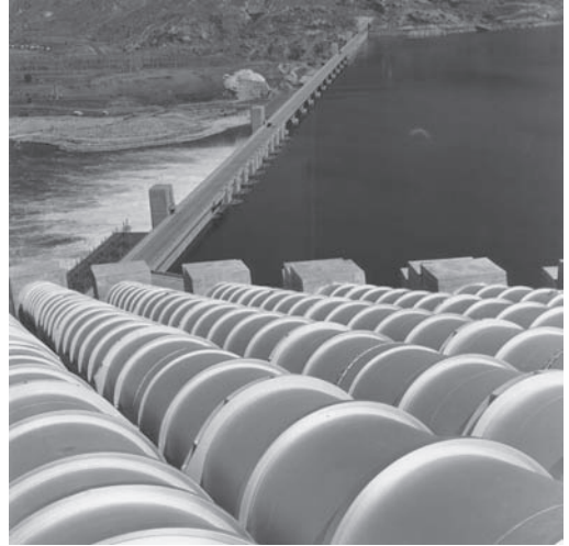
irrigation Huge irrigation pipes scale the walls of the Columbia River Gorge at Grand Coulee Dam, carrying water from the reservoir behind the dam.
