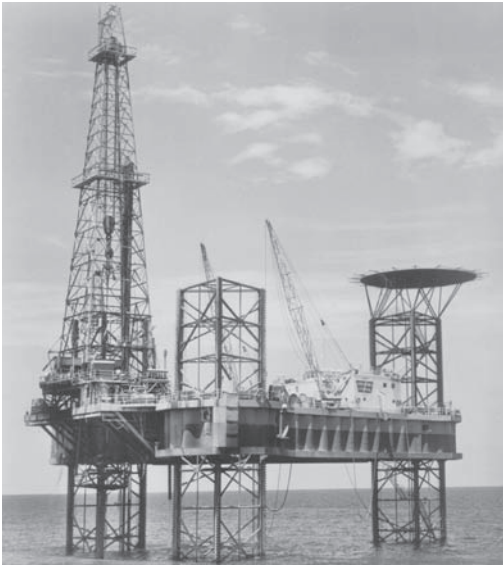
offshore Offshore drilling rig in the Gulf of Mexico, including a helicopter port and platforms that can be raised or lowered.
