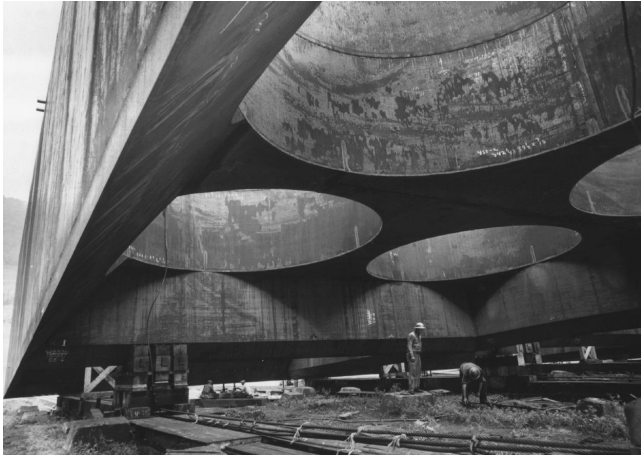
Underside of open caisson for Greater New Orleans bridge over Mississippi River. (Dravo Corp.)
