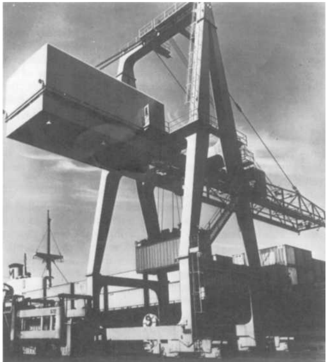
Container crane and straddle carrier.
