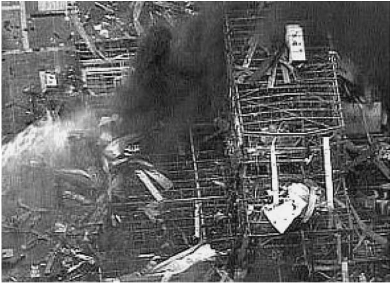
Figure 3-11 Aerial view of West Pharmaceuticals explosion residual fire.
