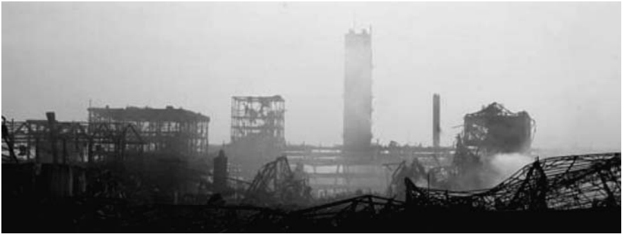
Figure 1-1. Aftermath of September 21, 2001 ammonium nitrate explosion in Toulouse (from UNEP APELL web site).
