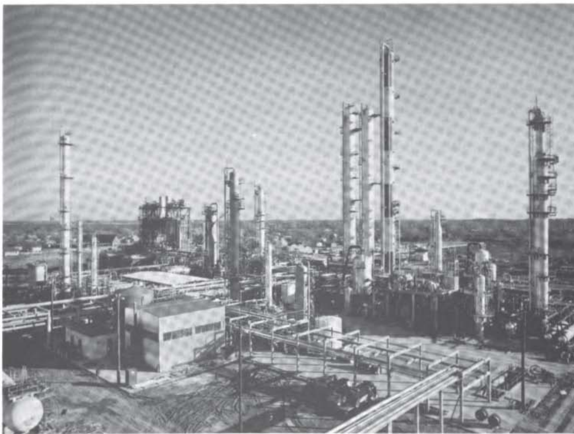
Figure 13-29 A panoramic view of the Sinclair-Koppers 230 million kilogram per year ethylene plant built by Pullman Kellogg at Houston, Texas. The pyrolysis furnaces are the rectangular units in the far left background. The tall tower at the right is the demethanizer. The tallest tower, painted in two colors, is the C_2 splitter. Just to the left of it are two large towers which compose the C_3 splitter, operating in series. (Pullman Kellogg, Inc., Houston, Texas.)
