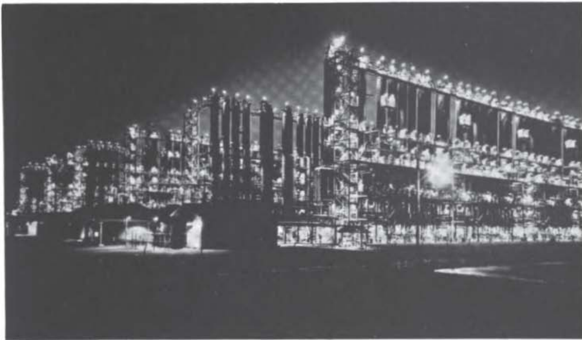
Figure 6-29 Countercurrent plate columns used for the manufacture of heavy water by hydrogen sulfide–water dual-temperature isotope exchange at the U.S. Department of Energy plant at Savannah River, South Carolina, ( The Lummus Co., Bloomfield, N.J. )
