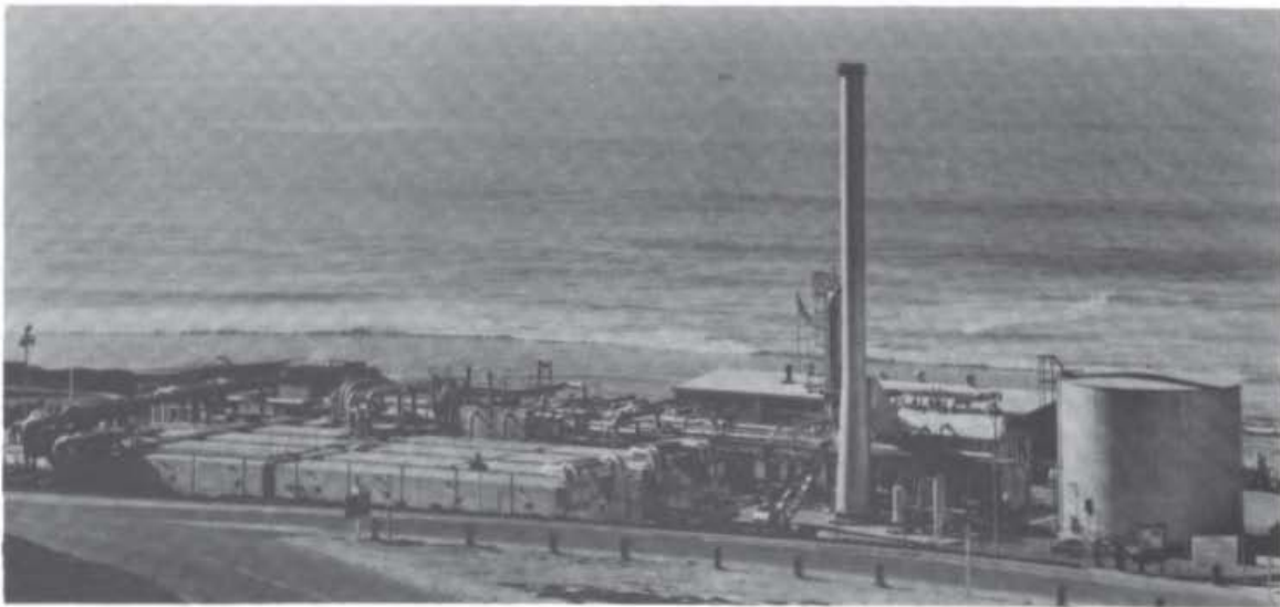
Figure 4-50 A multistage flash seawater desalination plant with a capacity of 3800 m 3 /day, originally located at Point Loma, California, and subsequently transferred to the United States Guantanamo Naval Base in Cuba. ( The Fluor Corp., Ltd., Los Angeles, Calif. )
