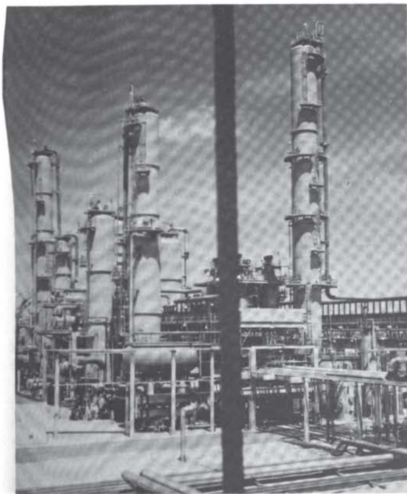
Figure 1-11 Distillation towers in the aromatics recovery unit at the Texas City, Texas, refinery of the American Oil Company. ( Pullman Kellogg Co. )
