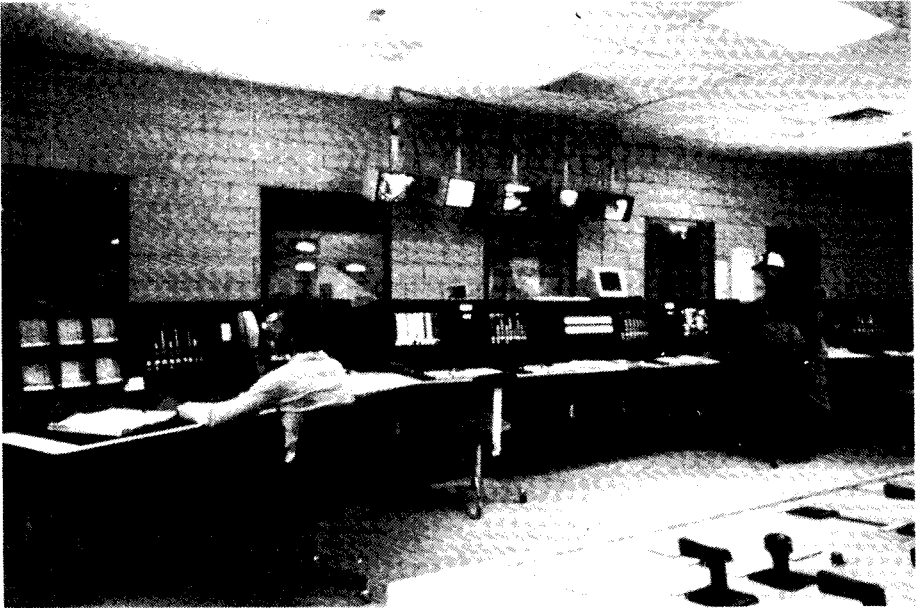
FIGURE A.9 Typical control room with computer control. (Courtesy of Honeywell.)
