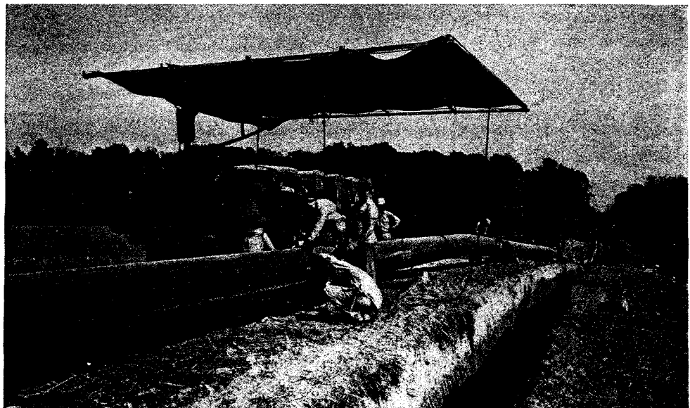
Fig. 17-7. Electric welding equipment. (Courtesy American Louisiana Pipe Line Company.)
