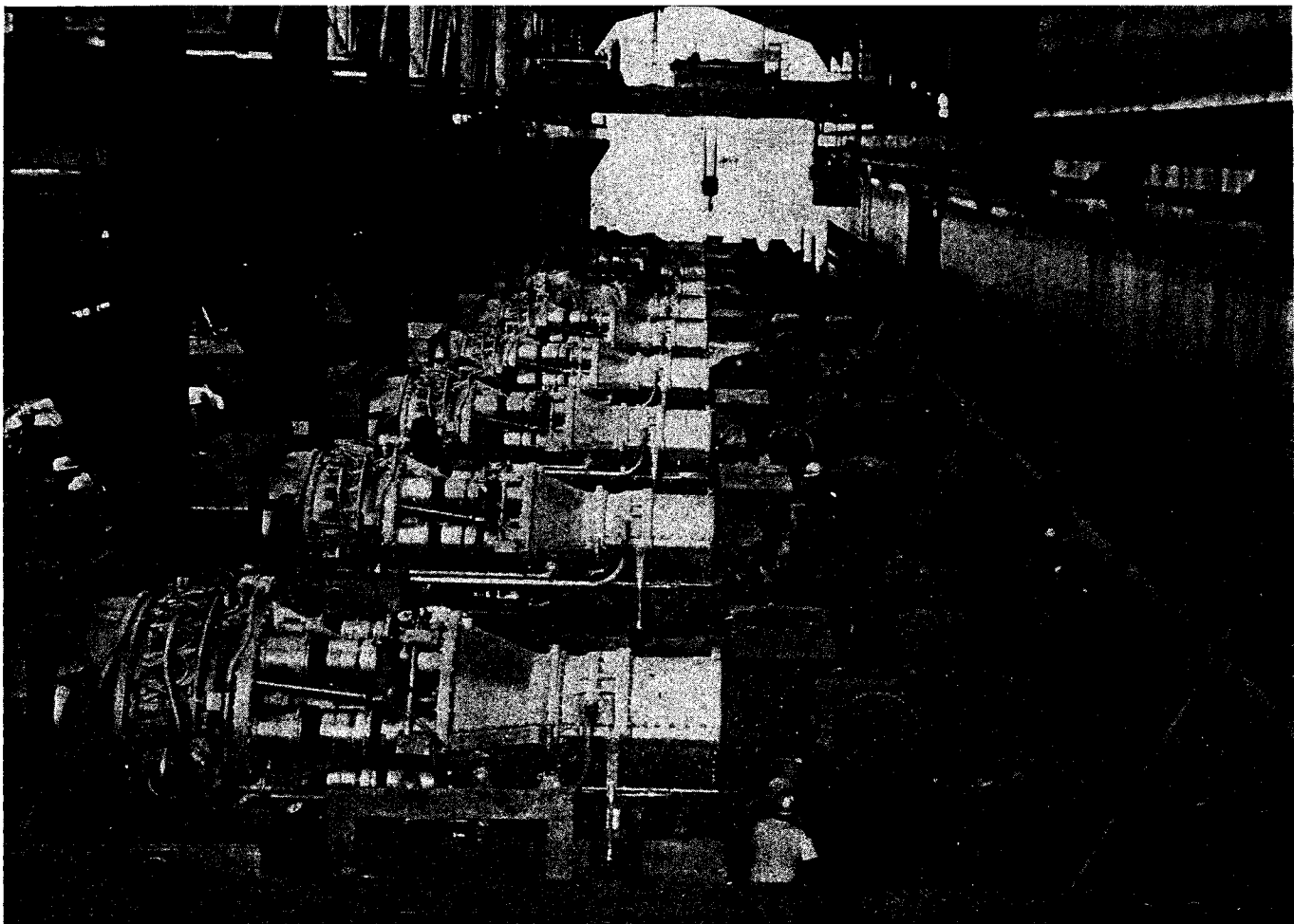
Fig. 17-22. Gas-turbine-driven centrifugal compressors. Ten gas turbines, 6,000 hp each, at Lake Maracaibo. (Courtesy General Electric Company.)
