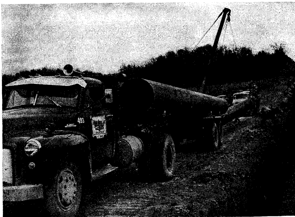
Fig. 17-3. Truck with pipe trailer for stringing pipe. (Courtesy H. C. Price Company.)
