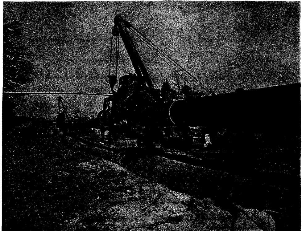
Fig. 17-9. Coating and wrapping machine. (Courtesy American Louisiana Pipe Line Company.)
