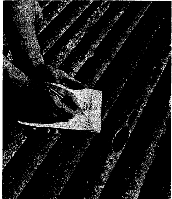
Fig. 11-36. Corrosion in tubing from gas well in North Markham field, Tex. (Courtesy Ohio Oil Company.)
