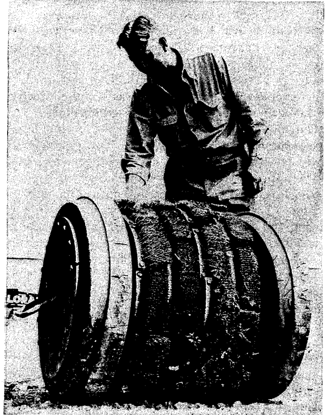
Fig. 17-16. Pig for cleaning pipeline.
