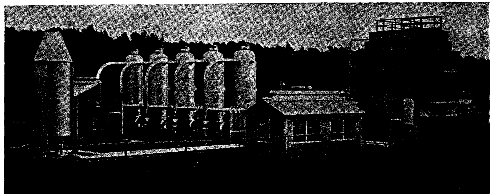
Fig. 18-11. Dehydration plant: solid desiccant; capacity, 240 MMcf/day; operating pressure, 650 psig.
