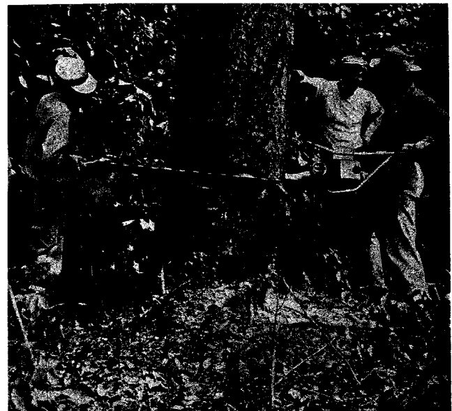
Fig. 17-1. Chain saw for clearing right of way. (Courtesy H. C. Price Company.)
