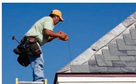
▲ Slate is not porous. It is made up of layers, so it can be split into thin sheets. This is why it makes good roofing tiles.
