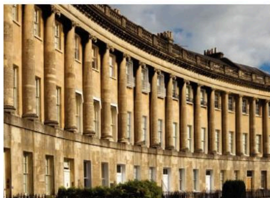
▲ Limestone is made from shells and skeletons that sank to the bottom of the sea. It is an attractive building material.
