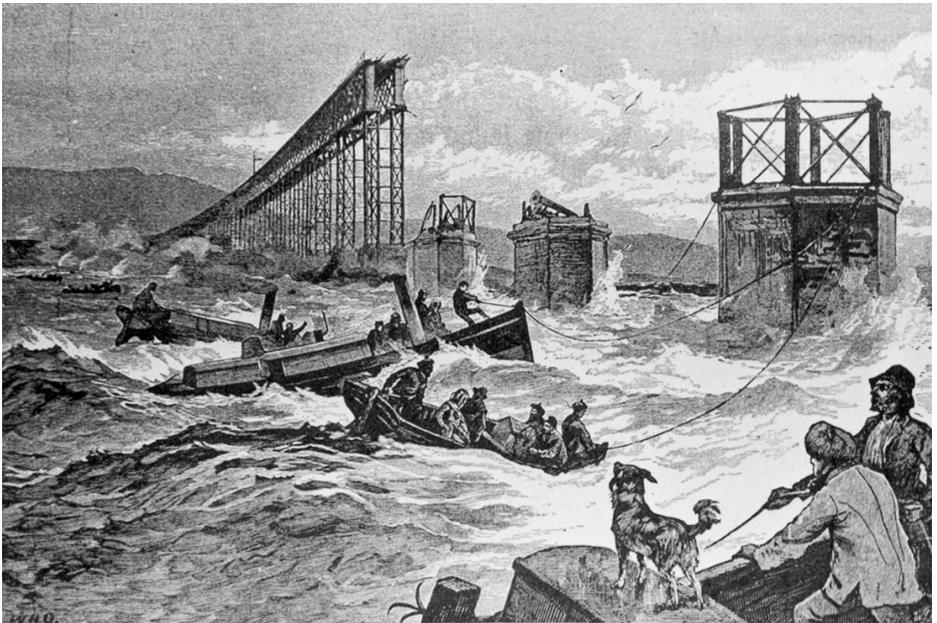
Cheap steel from the Bessemer process encouraged engineers to use it for large structures, usually successfully; but the rail bridge over the river Tay failed in high wind in 1879, costing the lives of 73 train passengers.
