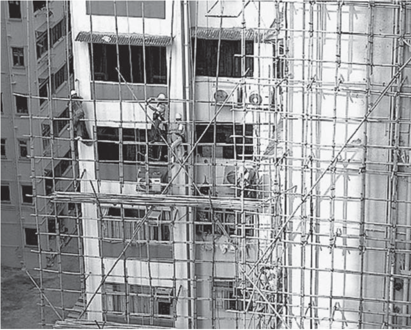
Bamboo scaffolding being used to construct a skyscraper in Hong Kong.
