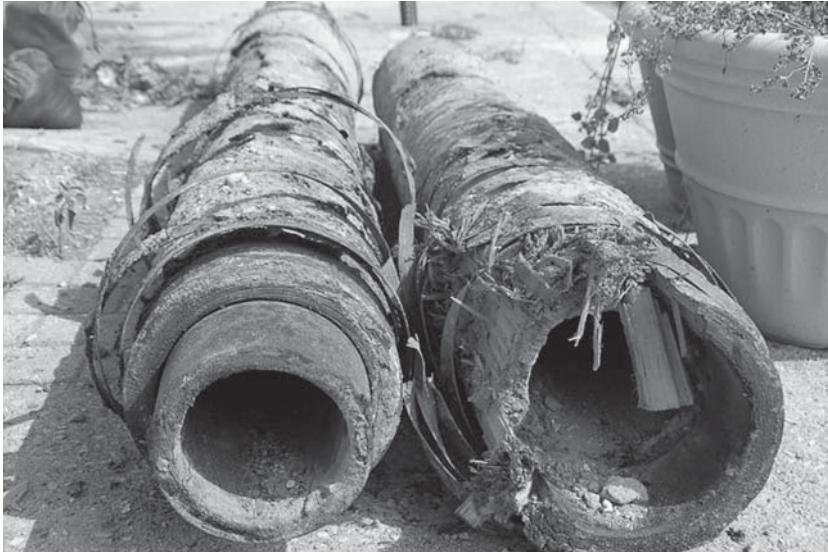
Two sections of 120-year-old wood pipe unearthing in Holly, Michigan, in 2007. In Detroit, 50 miles away, over 22 miles of wood pipe have been unearthing.
