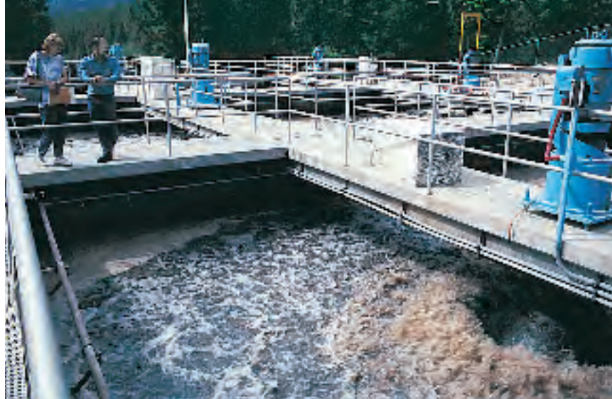
Figure 10 Air is bubbled through the sewage in this aeration tank so that bacteria can break down much of the sewage wastes. Determine whether the bacteria that live in this tank are aerobes or anaerobes.
