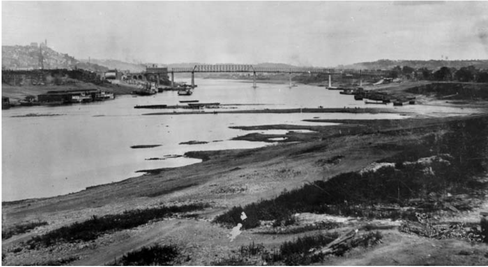
Figure 5.5 The Ohio River at Cincinnati, Ohio (approximately 1888), before impoundment. Photo was taken at low water, showing presence of shallow shoals and gravel bars. Note people on gravel bars in the distance for scale. From the collections of The Public Library of Cincinnati and Hamilton County, and the Cincinnati Historical Society Library.
