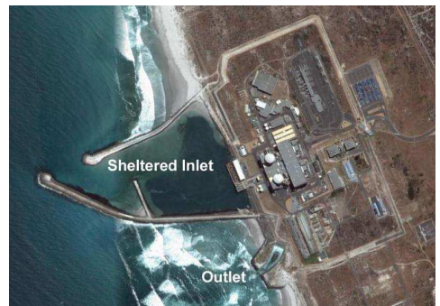
Aerial photo of Koeberg Power station
