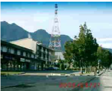
This tower was the culprit
