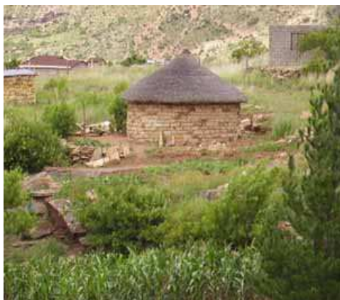
Round hut in nicely dressed stone masonry
