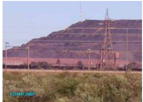
Giant iron ore mine near Sishen - Note the towers on top of the dumps
