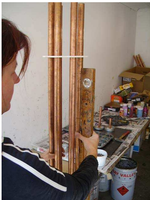
Make sure the pipes are level
