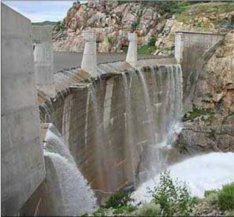
Overflowing Swakoppoort Dam (Photo: AZ Windhoek)
