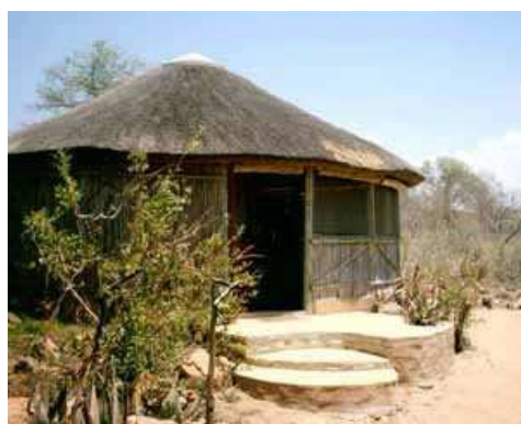
Sleeping hut, done in a simple gum pole and thatch construction but with great taste and attention to detail
