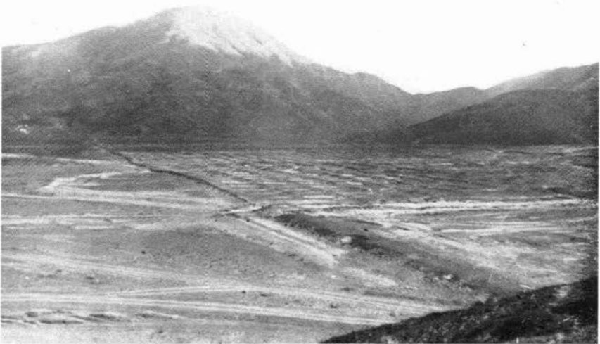
FIG. 79. The ancient civilizations of Peru had skilled engineers. In the upper view is seen one of the ancient aqueducts still intact for thirty-five miles which modern scientists estimate was capable of delivering sixty million cubic feet of water per day. They had no hardened tools or blasting powder, yet they cut this channel through boulders and rocks. Below is seen a valley covering thousands of acres once made fertile by irrigation but now an arid desert.
