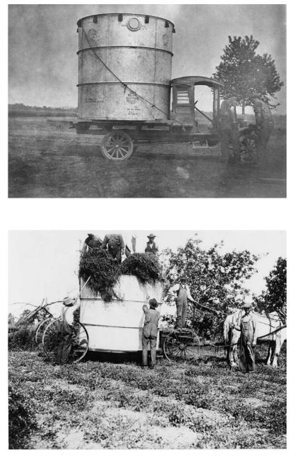
FIGURE 6.4 Examples of the tub (trailer still) designs that have been used in the United States over the years.
