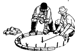
Make a mold for the slab.
