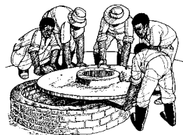
Set the well cover in place.
