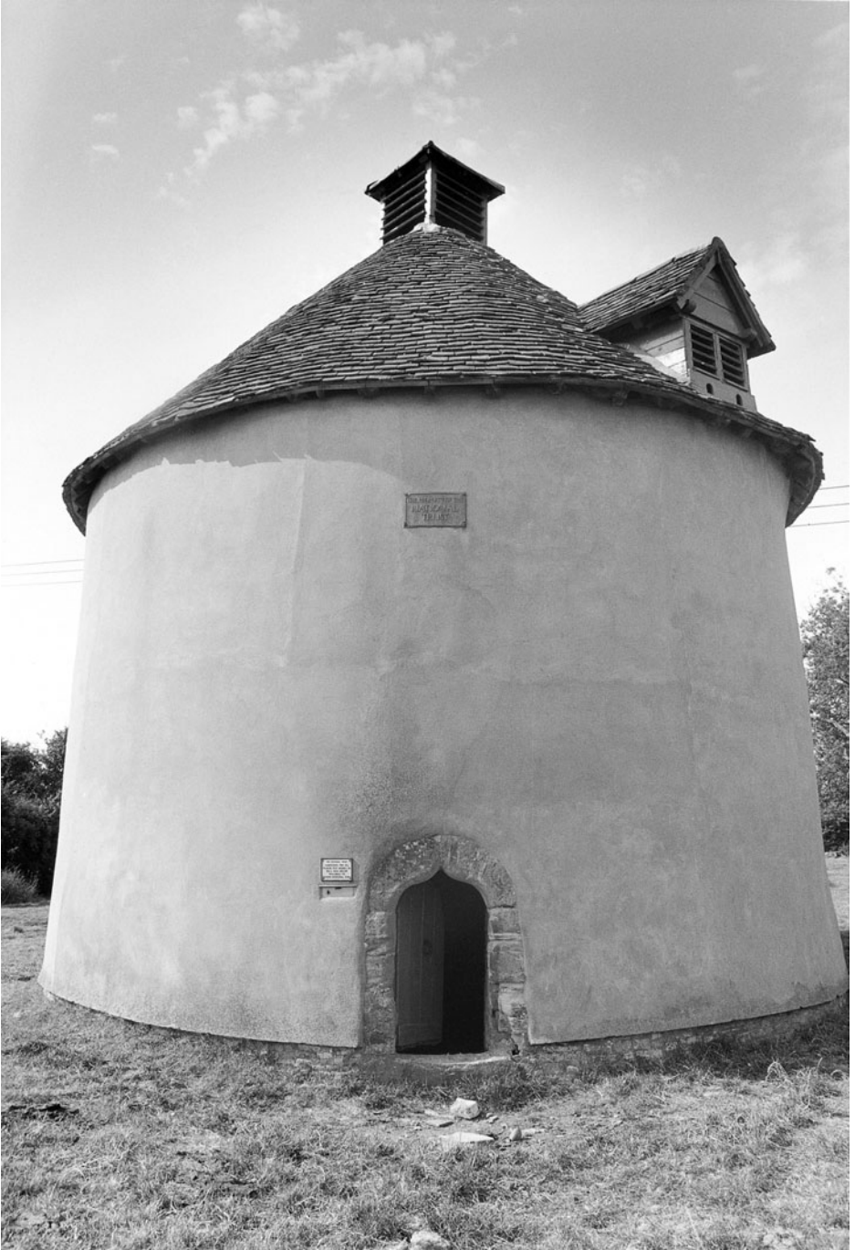
Plate 14.1 The fourteenth-century dovecot at Kinwarton in Warwickshire, built for Evesham Abbey. It contains 600 nesting holes. Inside the wooden device for supporting a rotating ladder survives. This gave ready access to the nests, enabling young birds to be taken for the table. Photograph: © William Muirhead and the National Trust.
