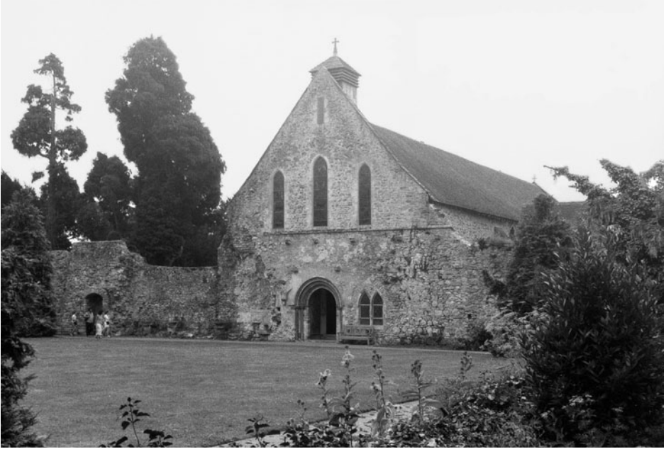
Plate 7.2 The refectory of Beaulieu Abbey, on the south side of the cloister, early thirteenth century, now Beaulieu church. Photograph: C. M. Woolgar.
