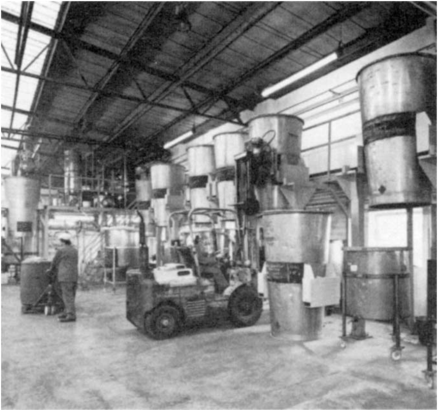
Figure 2–2 Solvent extraction plant.
