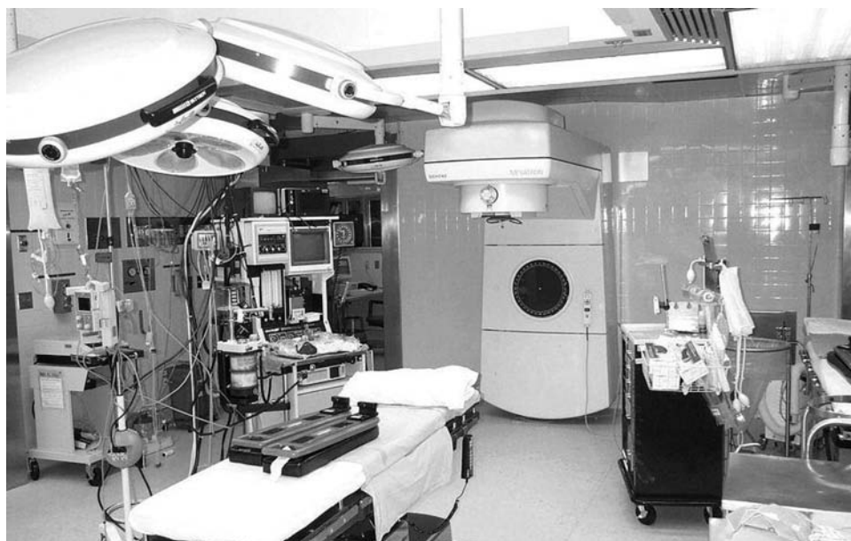
Figure 4. Mevatron ME by Siemens Medical Systems located in an OR. Note that the machine is a conventional accelerator whose gantry (C-arm) support system is mounted in the end wall. Since the room is slightly oversized for an OR room at this hospital, this still leaves adequate room for surgery.
