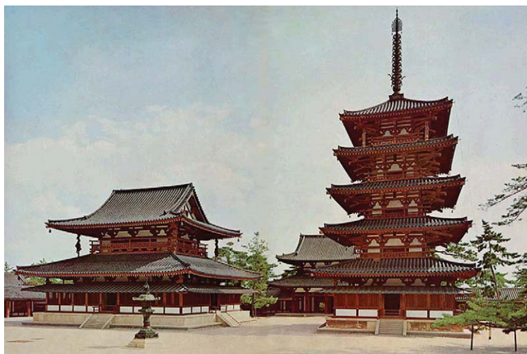
Figure 50 The Horyu-ji temple in Ikaruga (Nara Prefecture), Japan. On the right is the Gojunoto (five-story pagoda) and on the left, Kondo (main hall). Most of the temple buildings are built with Hinoki cypress ( Chamaecyparis obtusa ). Through dendrochronological analyses it was estimated that the trees used for the construction of the pagoda and the main hall were felled in 594 and between 667 and 669, respectively. Photograph from Shogakukan Inc., Tokyo, Japan.
